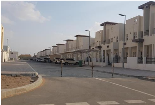
Figure 2: MREIFA Compound, Pedestrian Entrance
