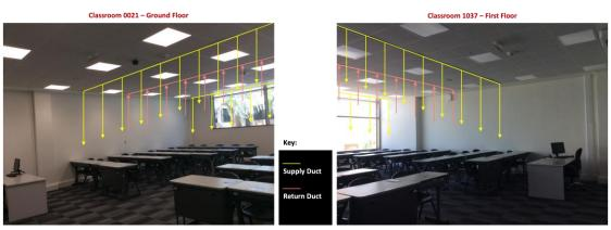
Figure 20: Showing the Supply and Return Air Ducts in Three Classrooms
