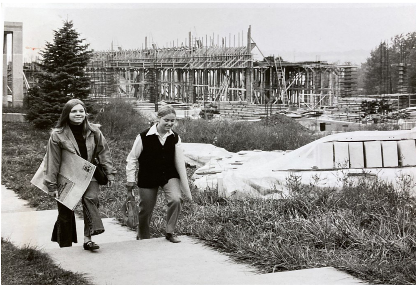
Art students Susan Ehman and Sandy Budd walked outside Sharadin and in front of construction for the new fine arts addition.
