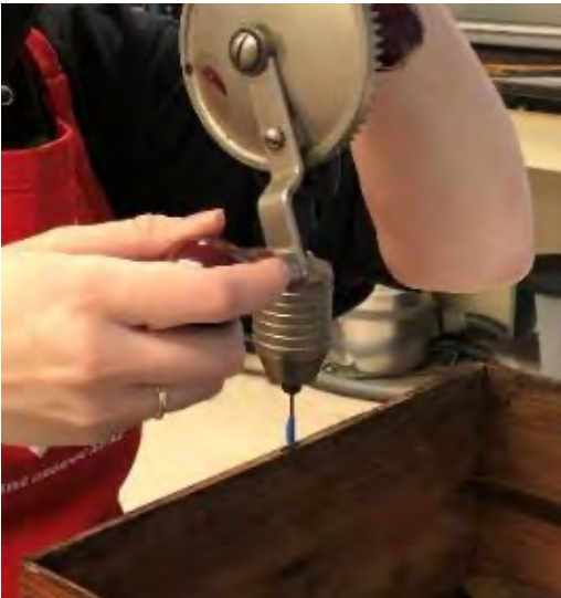
Fig. 20. Drilling out the tenon fragments from the mortises on the underside of the cabinet with a hand drill to make room for new tenons, to provide a more structurally sound joint during subsequent re-assembly.
