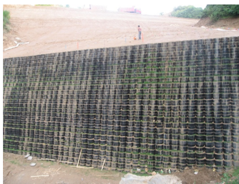
(b) Photo of geocell reinforced retaining wall
