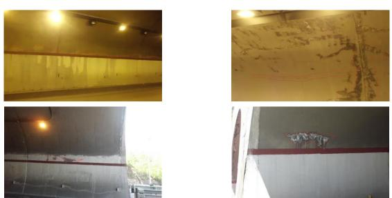
Fig. 3 - Vertical linear water seepage
