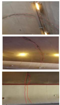
Fig. 2 - Circular linear water seepage
