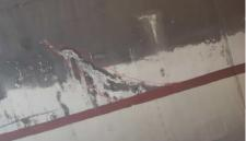
Fig. 4 - Slant linear water seepage
