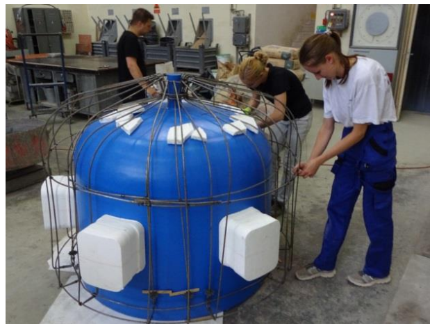
Fig. 8 – Assembly of reinforcement on the inner mold in the laboratories of the Faculty of Civil Engineering CTU in Prague.
