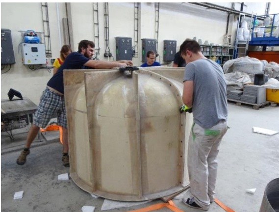
Fig. 9 – Fitting the outer mold part (Laboratory of the Faculty of Civil Engineering, CTU)
