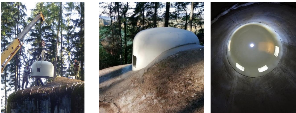
Fig. 18 – Placement of the replica and realization of concreting (pillbox T-S 20)
