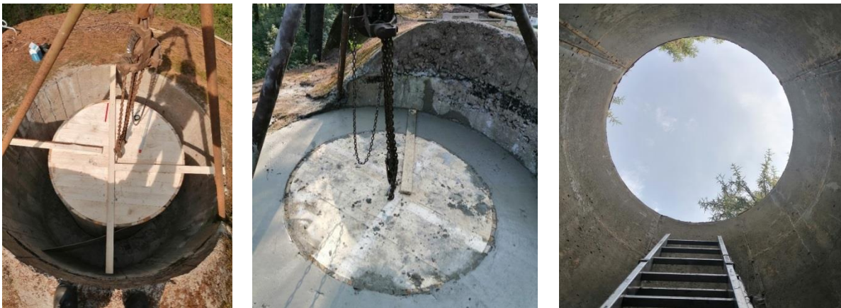
Fig. 17 – Realization of the lower monolithic part of the cloche (pillbox T-S 20)
