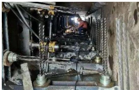
Fig.5-1 Picture of working steel pipe of bundled integrate structure
