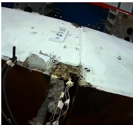
Fig.3-3 Initial state of No.2 seam section
