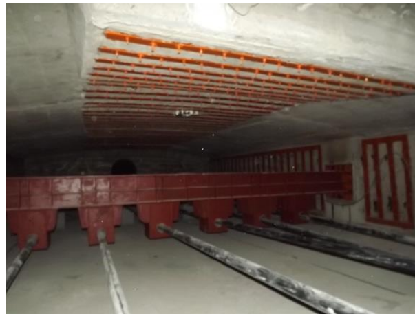
Fig.6 - Field condition of external prestressed bundle
