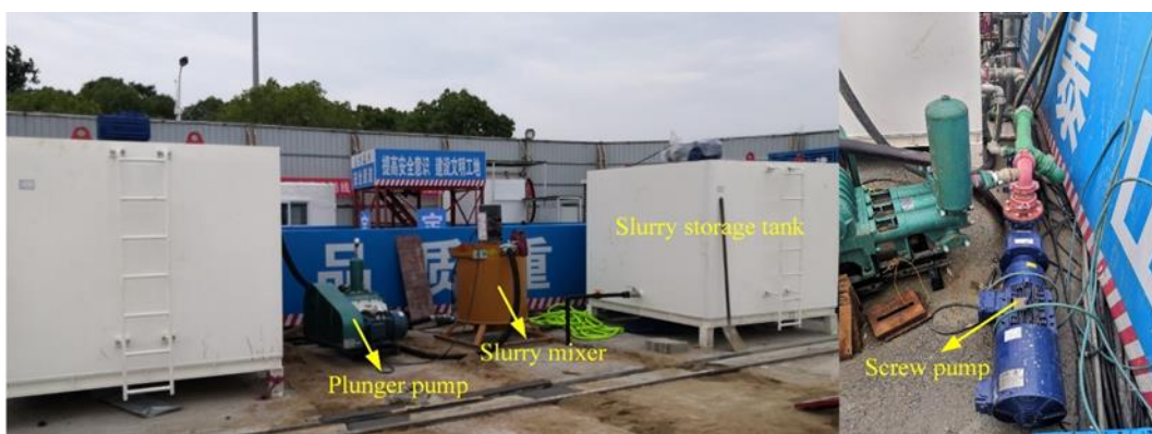
Fig. 6 – Layout of thixotropic slurry system
