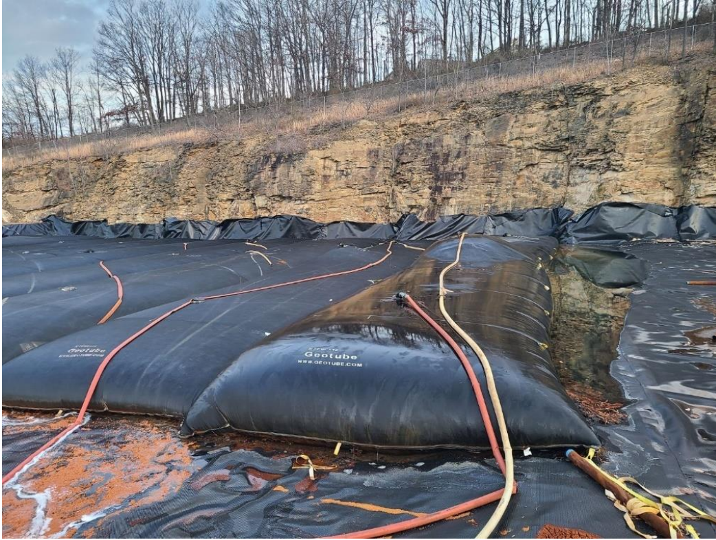
Figure 1: Geotextile tubes dewatering (Source: Tyson 2022)
