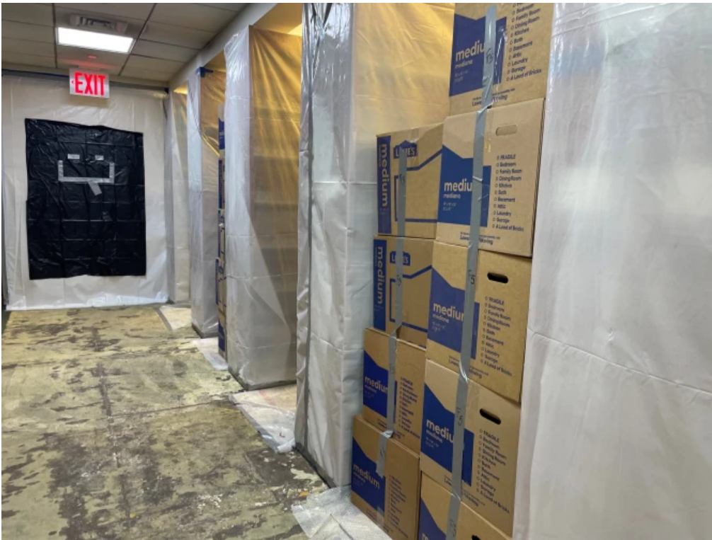
Part of the library's construction zone.
