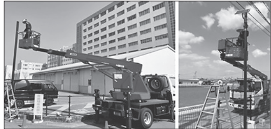
Fig. 2 State of construction during the device installation
