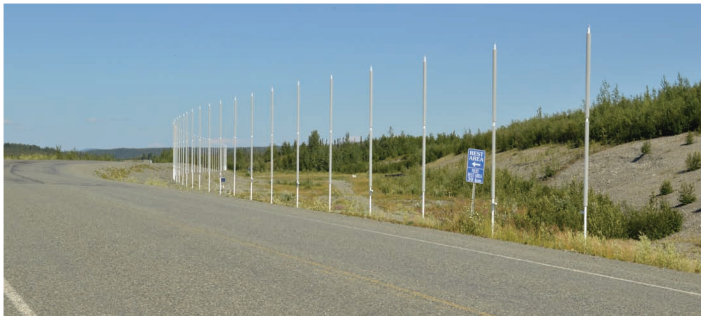
FIG. 12. Thermosyphons installed along the Alaska Highway at Dry Creek, YT (km 1840). These passive ground cooling installations are required to prevent a body of massive ice beneath the road from thawing. Photograph taken on 31 July 2021, © C.R. Burn.
