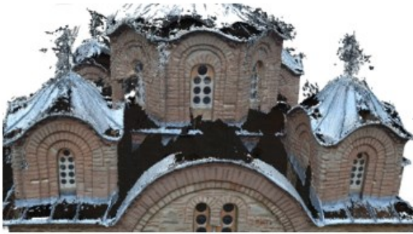
Figure 2. Terrestrial photogrammetry and the upper part of the church model.
