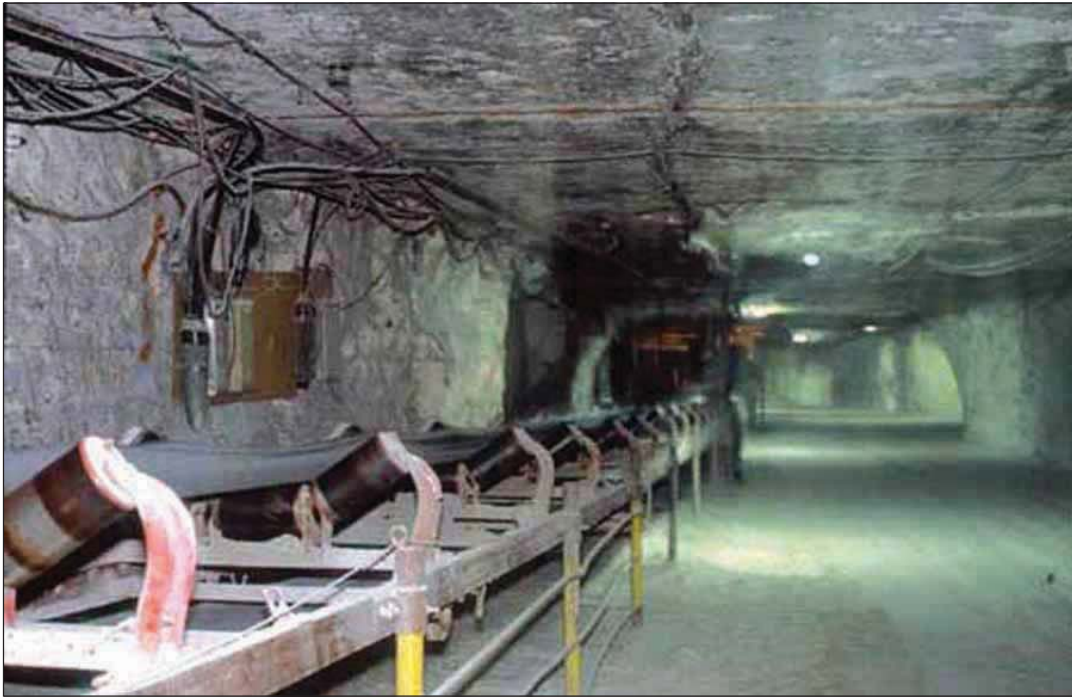
FIGURE 73—Room-and-pillar mining of salt at Hutchinson, Kansas; from Sawin and Buchanan (2002, p. 3, fig. 5).
