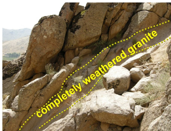
Fig. 5: Lying of instable blocks on completely weathered granite as basement.
