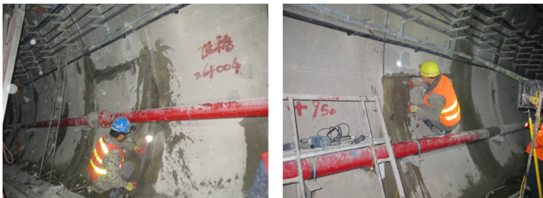
Fig. 10. Photos showing some the works of leakage treatment.
