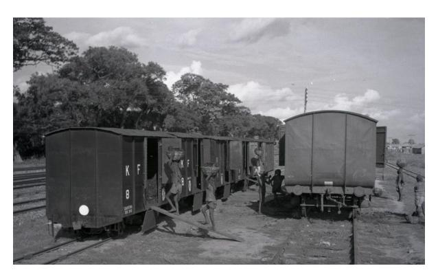
Image 2: Transferring coal from broad to narrow gauge 17
