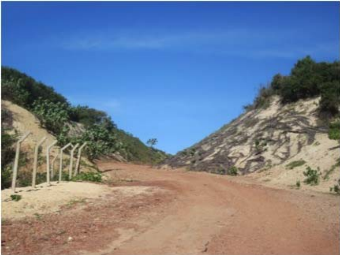
Picture 1. Dune compaction
