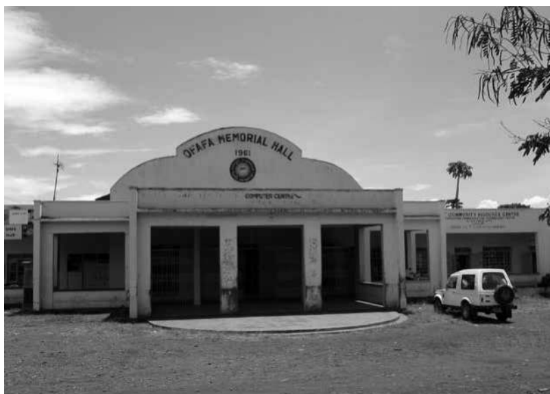
Figure 3.2. Ofafa Memorial Hall, Kisumu. Photo by author.
