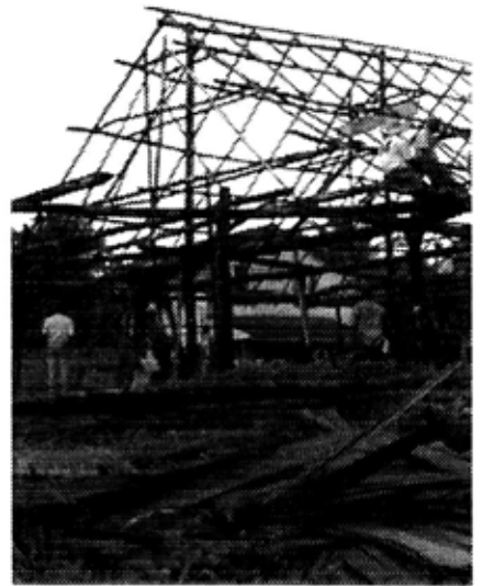
Men sit on the roof of the temple frame as they wait for the thatching to begin.
