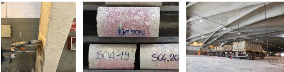
Fig. 17. Pavilion V: Extraction of concrete sample from a strut-beam (left); carbonation tests on sample of the ribs (centre); view of the static tests with trucks connected to the ribs through jacks (right).
