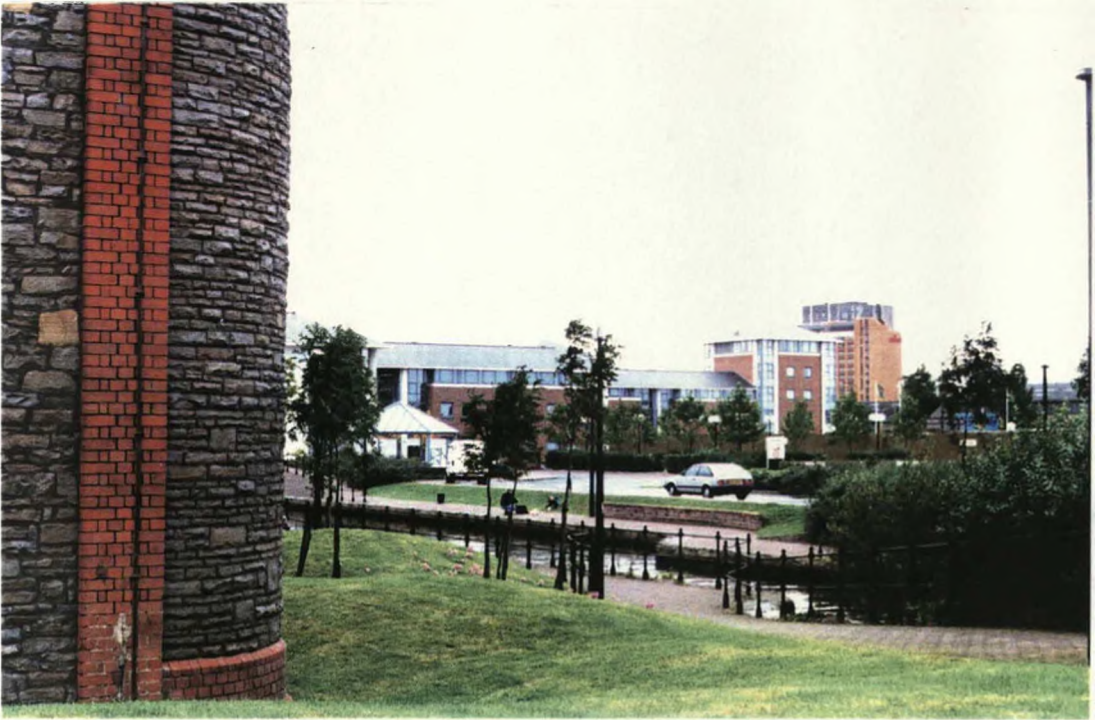
PLATE 4(6). Relationship between Tarmac's residential and commercial development, Atlantic Wharf, Cardiff, the Feeder canal, and development north of the canal (photograph, the author, 1992)
