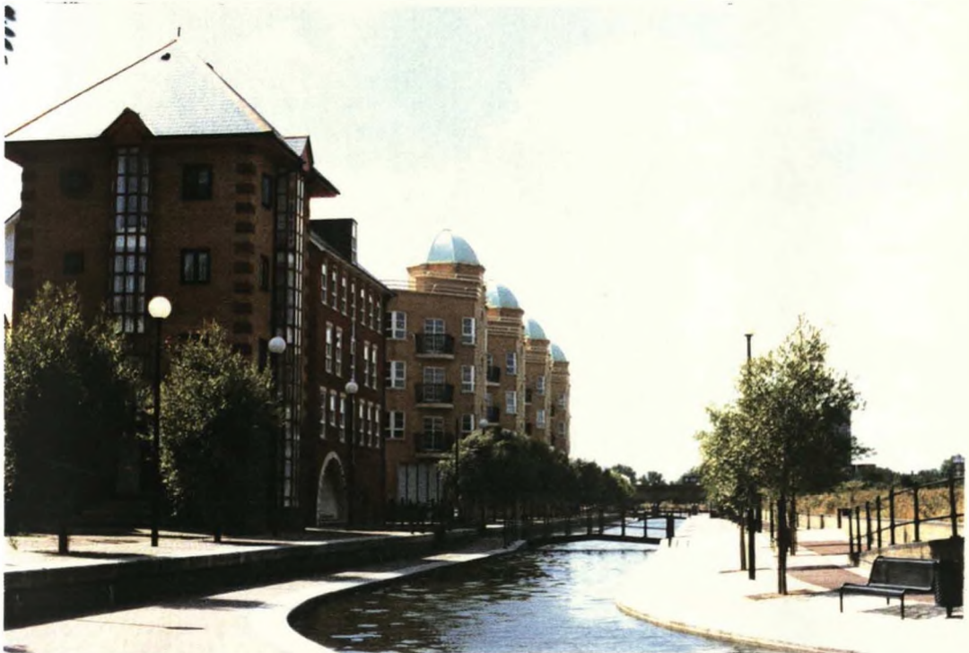
PLATE 6(2). Canalfront, Wolfe Crescent, Surrey Docks, London, considered to be "visually attractive" by the majority of questionnaire respondents (photograph, the author, 1989)
