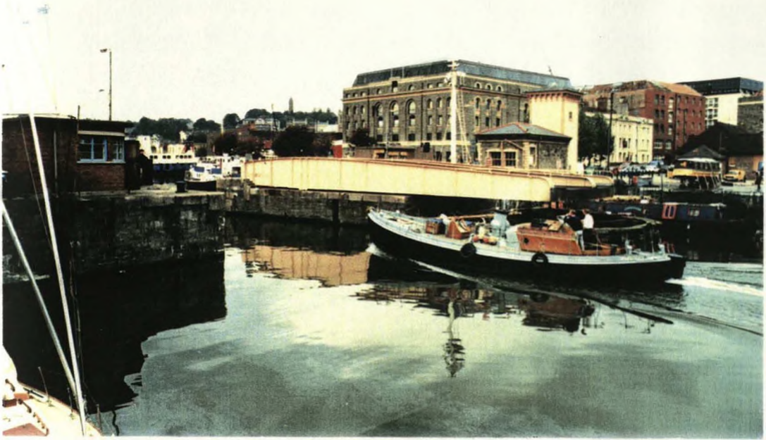
PLATE 3(7). Entrance to the Floating Harbour, Bathurst Basin, Bristol Docks (photograph, John Horn, 1991)
