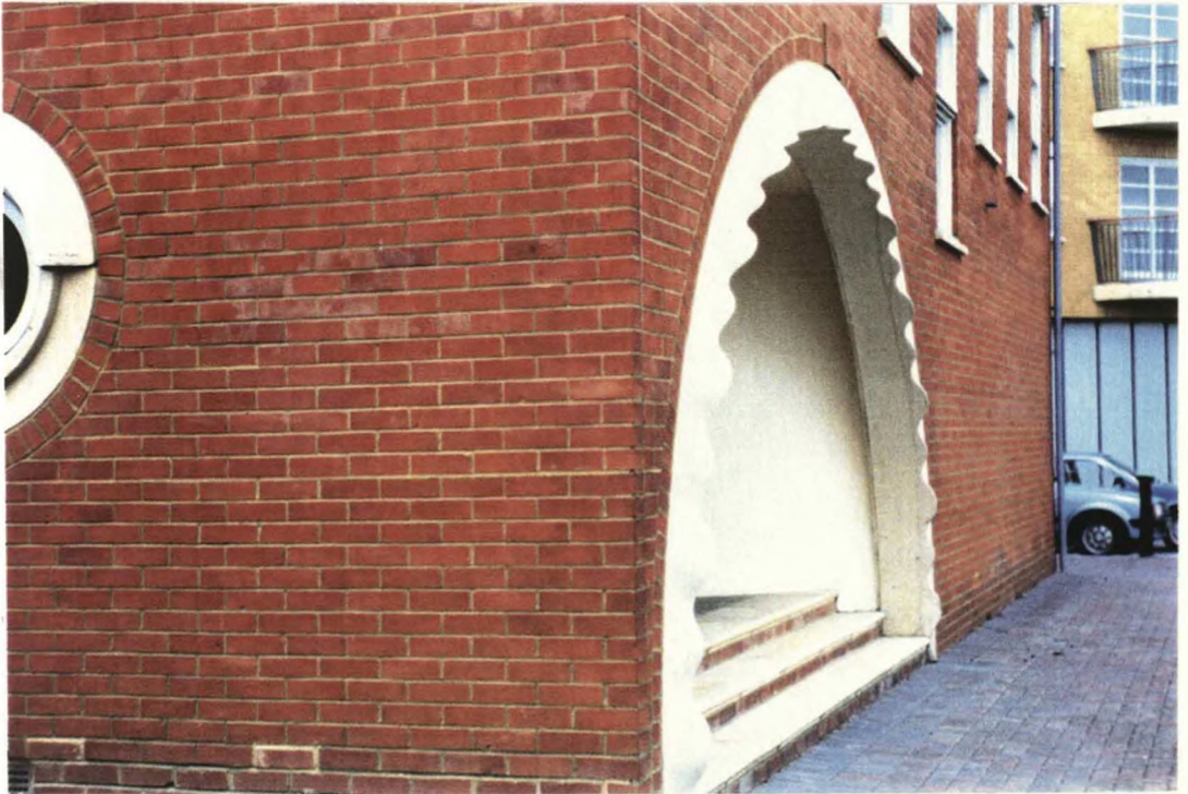
PLATE 5(3). Wolfe Crescent's pre-cast lintels, Surrey Docks, London, intended by Piers Gough (architect) to represent "raised curtains" (Jay Stuart of Campbell Zoogolovitch Wilkinson Gough, architects, personal communication). (Photograph, the author, 1989)
