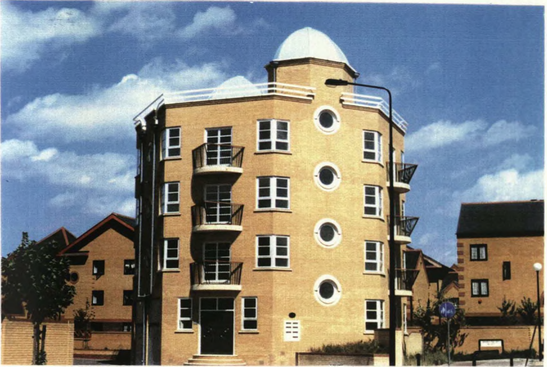
PLATE 5(2). Wolfe Crescent's octagonal towers, intended by Piers Gough (architect) to represent "players on a stage" (Jay Stuart of Campbell Zoogolovitch Wilkinson Gough, architects, personal communication). (Photograph, the author, 1989)
