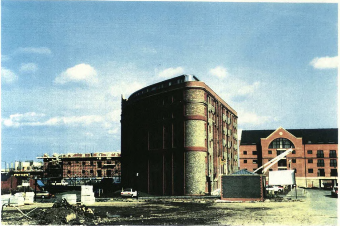
PLATE 4(13). Re-alignment of Tarmac's residential and commercial development, Atlantic Wharf, Cardiff; the developers' response to a request by the Royal Fine Arts Commission (acting on behalf of the Cardiff Bay Development Corporation) in 1987 to "recognise" the entrance of the Spillers and Bakers warehouse (photograph, the author, 1992)
