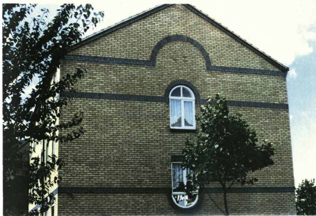
PLATE 5(12). Mirror glass window added to Lovell Urban Renewal's Marlow Landings development, Surrey Docks, London (photograph, the author, 1990)
