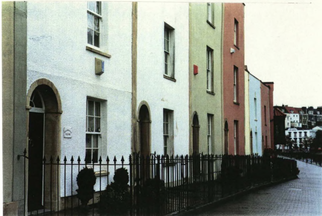
PLATE 4(17). Refurbished façades of nos 4-9 Bathurst Parade, Merchant's Landing, Bristol Docks (photograph, the author, 1992)
