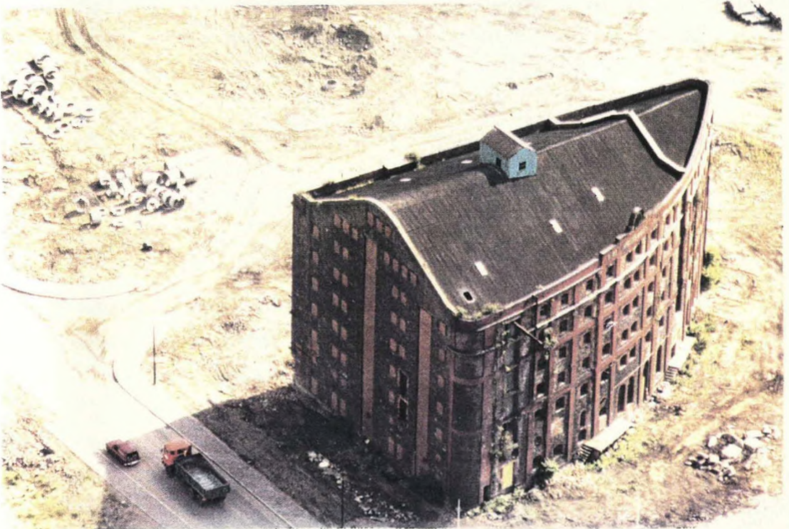
PLATE 3(4). Spillers and Bakers warehouse (1893-1987), Atlantic Wharf, Cardiff, prior to refurbishment (reproduced from Lovell, n.d.)
