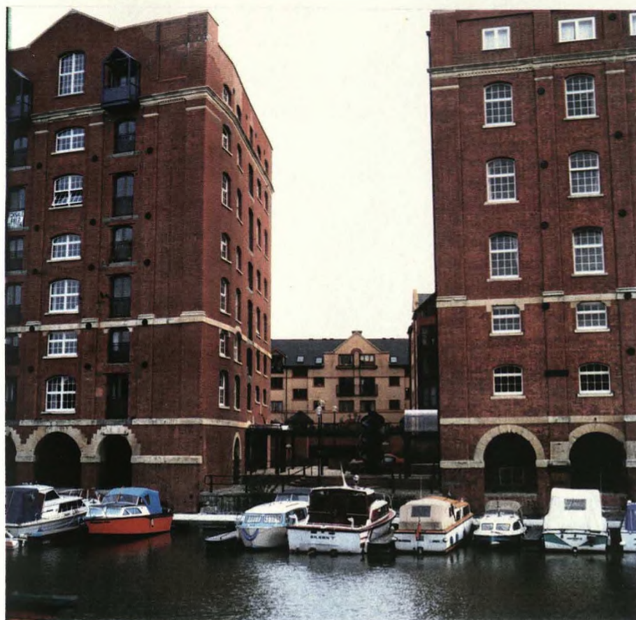
PLATE 4(15). Refurbished Buchanan's warehouses, Bristol Docks (photograph, John Horn, 1991)
