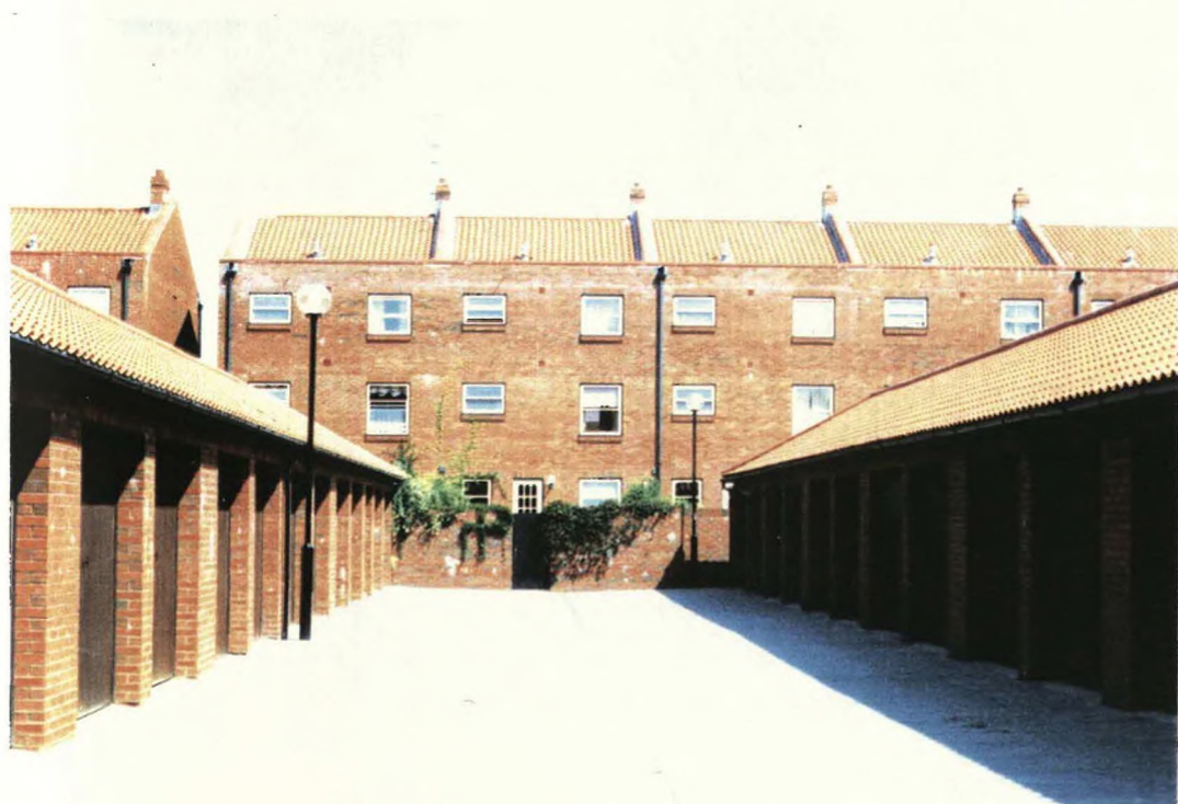
PLATE 4(18). Challoner Court garages, Merchant's Landing, Bristol Docks (photograph, the author, 1990)
