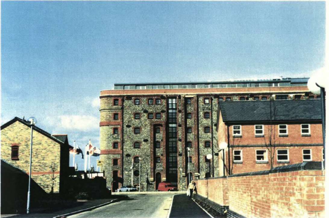
PLATE 4(14). Refurbished Spillers and Bakers warehouse, Atlantic Wharf, Cardiff, showing attic-roof extension (photograph, the author, 1990)
