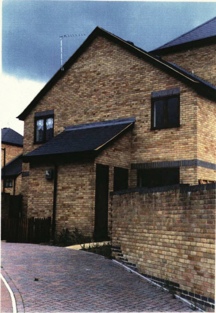
PLATE 4(3). Enclosure of end plots of Surrey Waters housing block "F", Surrey Docks, London, with a brick wall; the developers' response to a request by the London Docklands Development Corporation in 1984 to create a "clearer visual link" with Surrey Water (photograph, the author, 1989)
