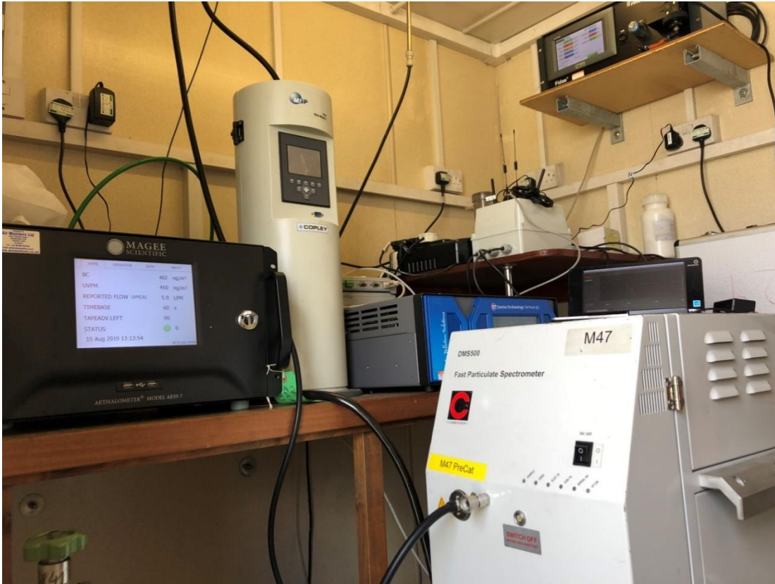
Fig S2: Instrumentation at LHR2. Clockwise from centre left: Magee AE33-7 Aethalometer, Nano-MOUDI cascade impactor sampler, Teledyne API T200 NO x analyser, Fidas 200 PM analyser, Cambustion DMS500 UFP analyser.
