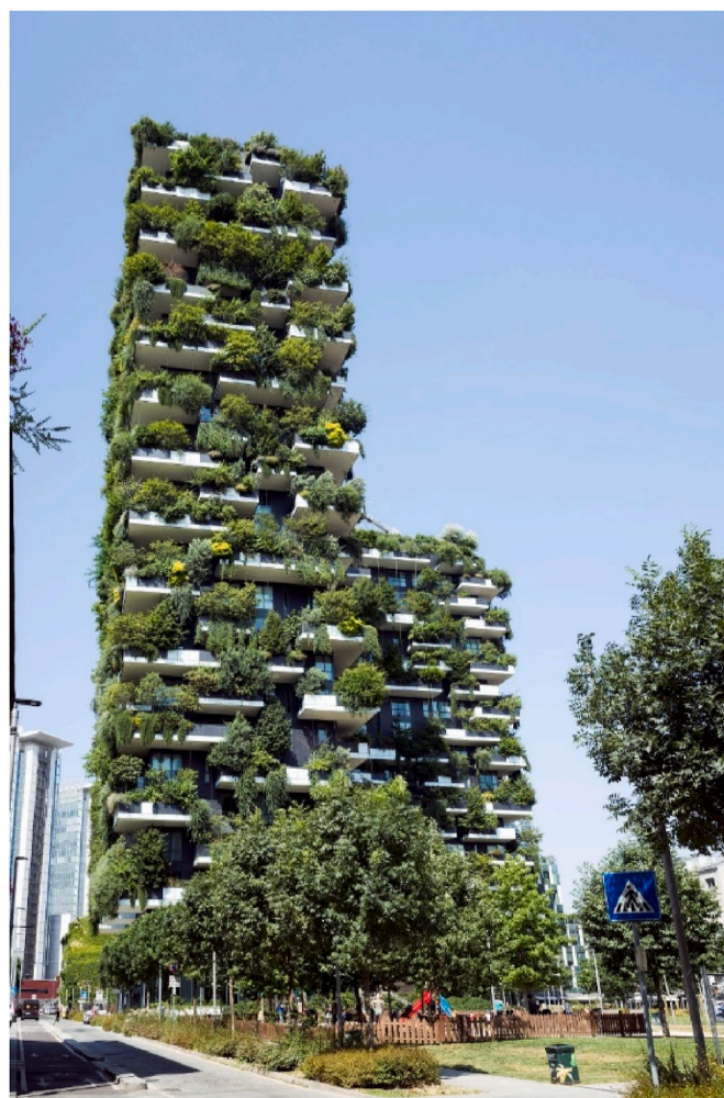
Fig. 2. Planted balconies of the Bosco Verticale. (Photograph by Andrej licensed under CC BY-NC-SA 2.0 [13]) ( https://www.flickr.com/photos/truu/42869769924 , Accessed 03.02.2022).
