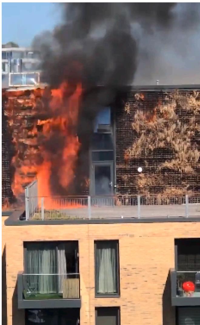
Fig. 3. Living Wall fire in London in 2018 (image is reproduced from video clip on twitter by @Miss_AnitaRaj 5 August 2018 [5]).
