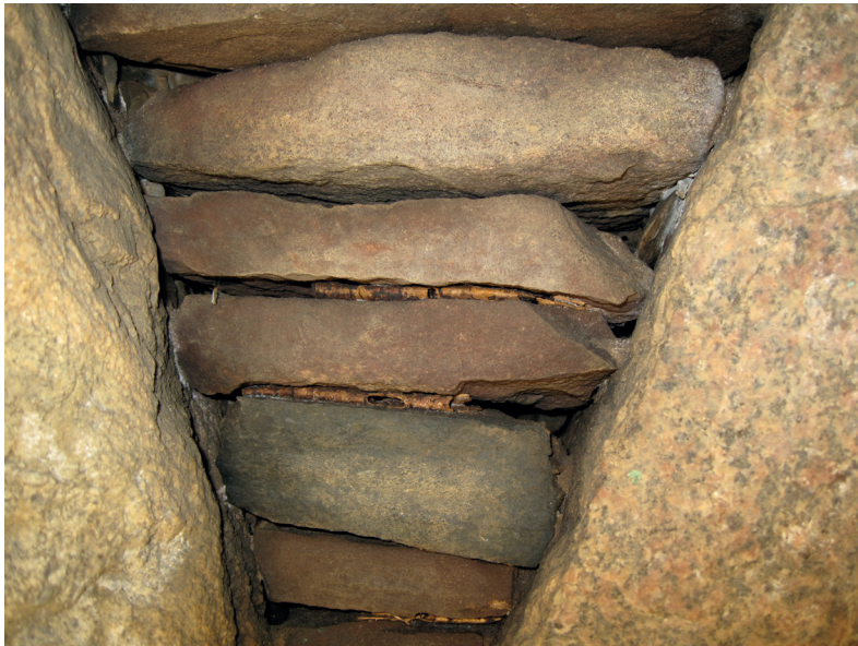
Figure 15. The folded birch bark between the sandstone slabs in the dry-walling in Maglehøj (Photo: L. Aa. Jensen, Danish National Museum).
