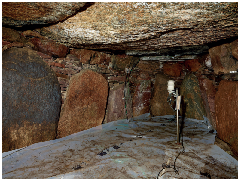
Figure 14. The Maglehøj chamber seen looking north, with a damp-proof membrane on the floor. The internal climate sensors can be seen on the right (Photo: R. Fortuna, Danish National Museum).
