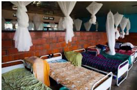
Image of hostel at University of Rwanda Campus where some improvements are still needed.
