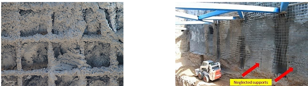
Fig. 2. Not completed shotcrete structures
