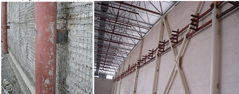
Fig. 6. Sudden change in the slenderness (left) and punching the columns and braces in order to pass the utility pipes (right)
