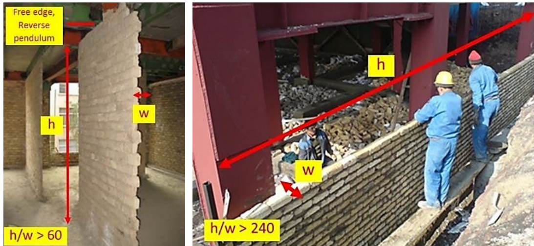
Fig. 5. Post-less slender walls
