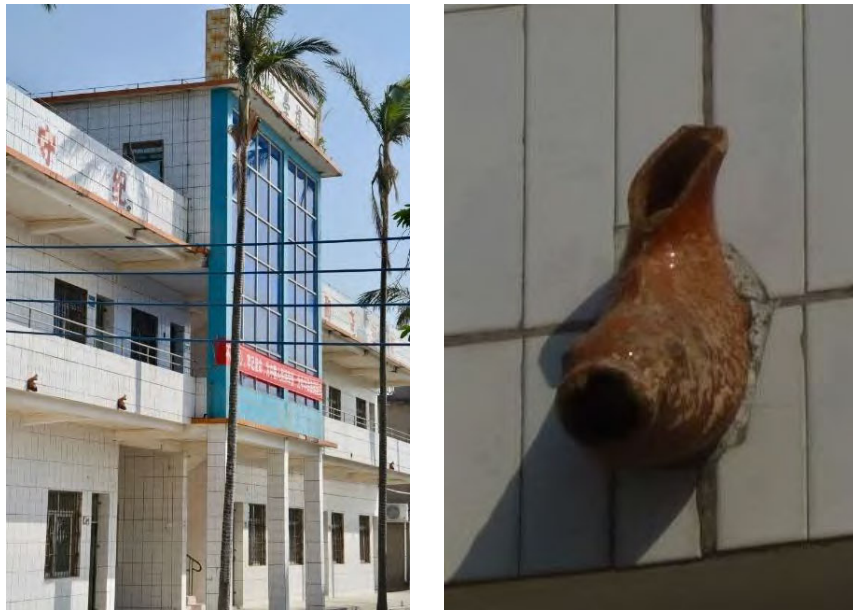
Figure 5.13 Façade of Sung-Sun Hall of Learning at Ma Shan School in Doumen, Zhuhai. (Photo by Denis Byrne, 18 December 2017.) On the right, a close-up image of the “fish-out-of-water” (鰲魚) rainwater sprout. (Photo by Christopher Cheng, 18 December 2017.)
