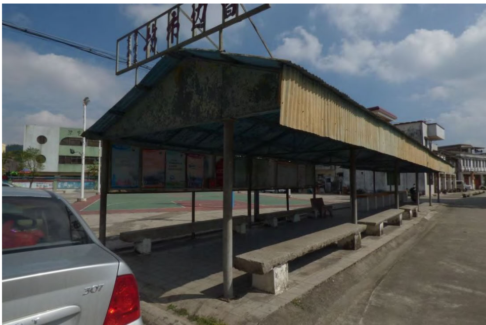
Figure 0.1 A shelter for the marketplace of Cho Bin village was built by Cho Bin emigrant and Townsville resident Philip Leong. The four-storey building, established in 1993 (the one with round windows behind the basketball court), was another of Philip’s initiatives. It was leased as a factory to provide long-term financial support to families left in the village. (Photo by Christopher Cheng, 2 December 2018.)
