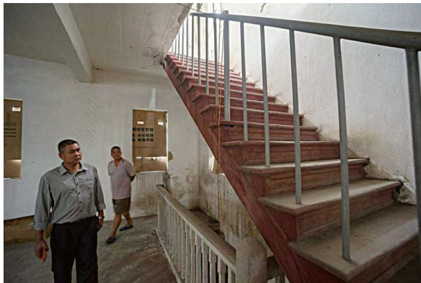
Figure 6.3 The new steel-tube handrails to the upper stories of Lai Wor School in Ngoi Sha village, Zhuhai, were reinstalled in the 1990s. (Source: Howard Wilson, private collection.)
