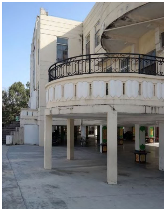
Figure 5.17 Heng Mei School in Zhongshan's South District was raised off the ground, creating a vast undercover activity space for its students. (Photo by Denis Byrne, 19 December 2017.)
