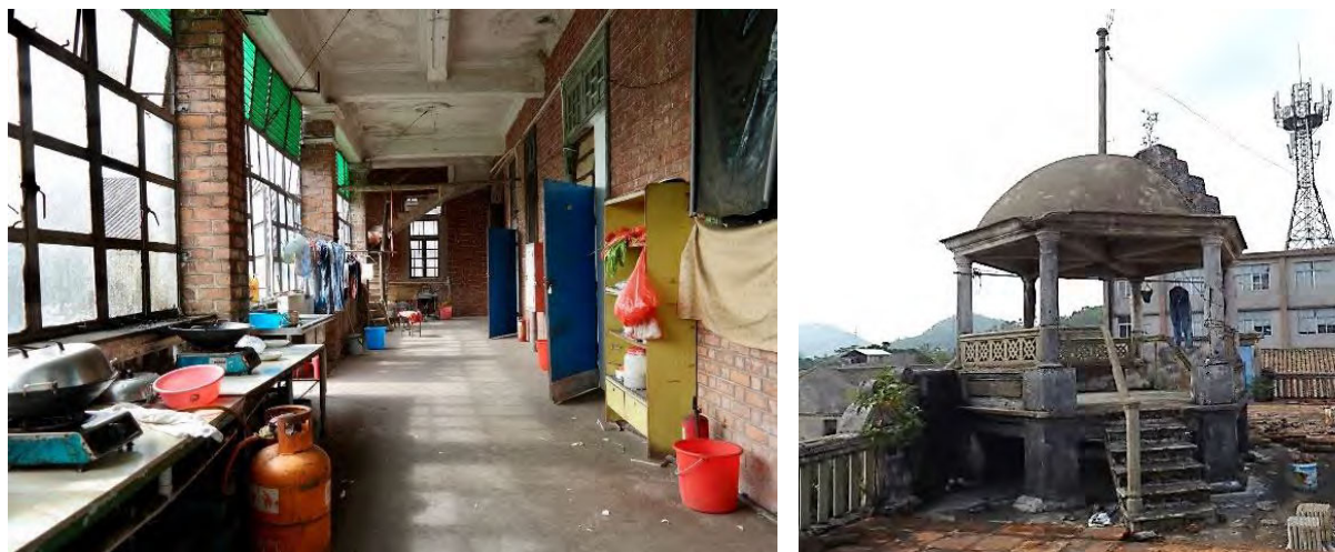
Figure 6.14 The infilled veranda (left) serving as the factory workers’ makeshift kitchen. (Photo by Denis Byrne, 2 December 2018.) The old school cupola (right), where the school bell once hung, had become a clothesline for resident-workers. (Photo by CHAN Yik-leung, 31 March 2019.)
