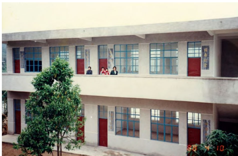
Figure 7.5 Chinese-Australian families return to visit the new donated kindergarten at Cho Bin village. The building was opened on 10 February 1987. (Photo by Joe Leong, 10 April 1988.)
