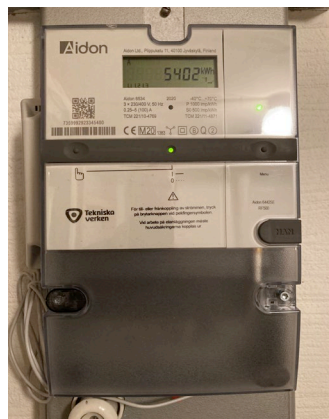
Picture 1. Example of a smart meter (photograph by one of the authors).
