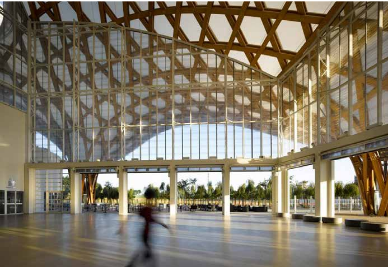
Fig. 5.24 Interior view of the Centre Pompidou Metz
