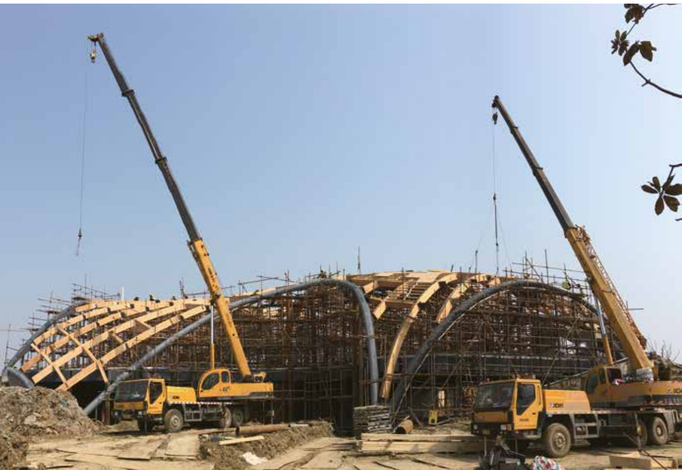
Fig. 5.26 Timber gridshell at Horticultural Expo Suzhou during construction
