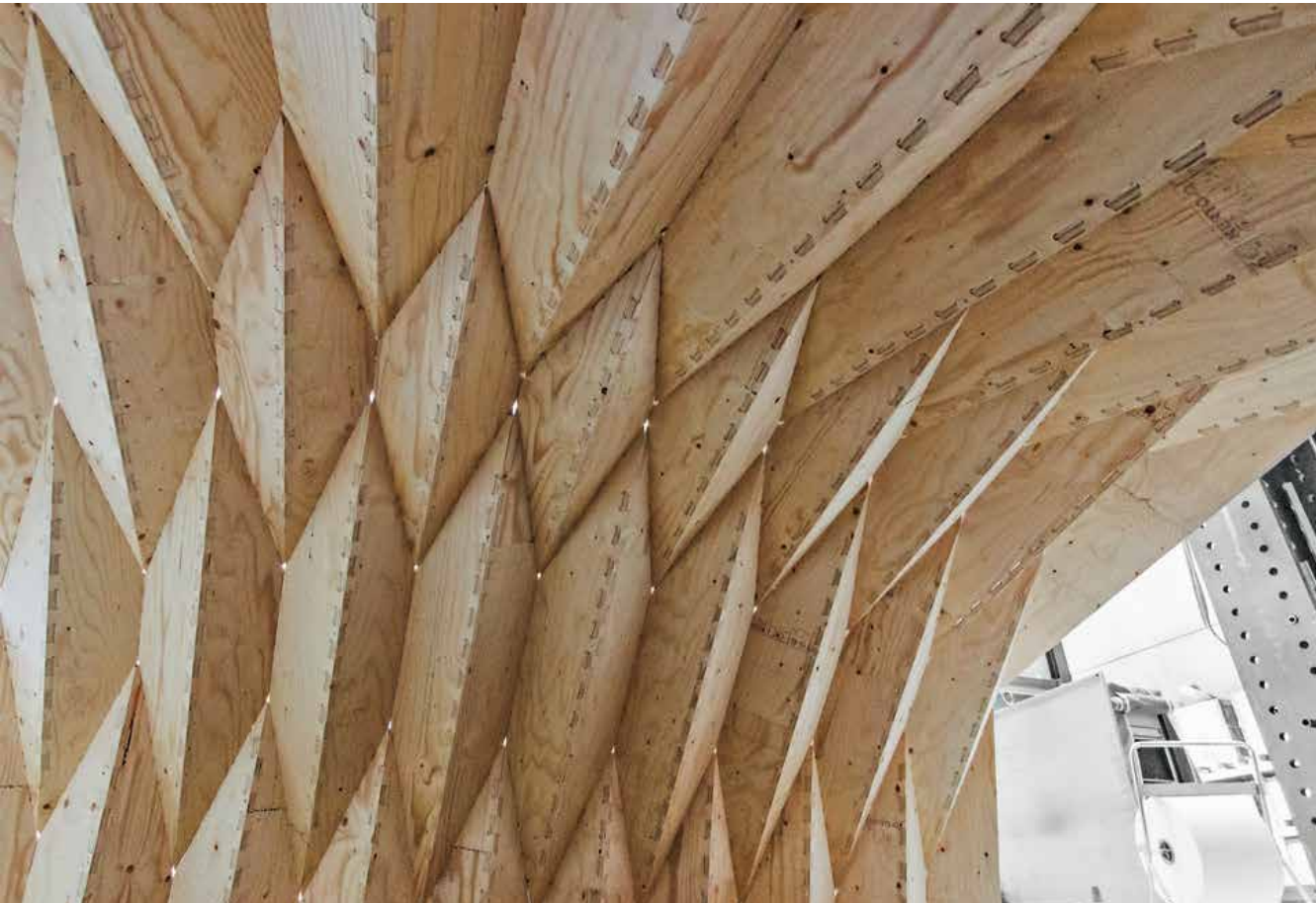
Fig. 5.29 Surface-active shell built at IBOIS as demonstrator for the structural resistance of timber forlidd plates and the related integral attachments in wood. The shell geometry is based on a slightly double curved arch and the connections are based on japanese dovetail finger joints.
