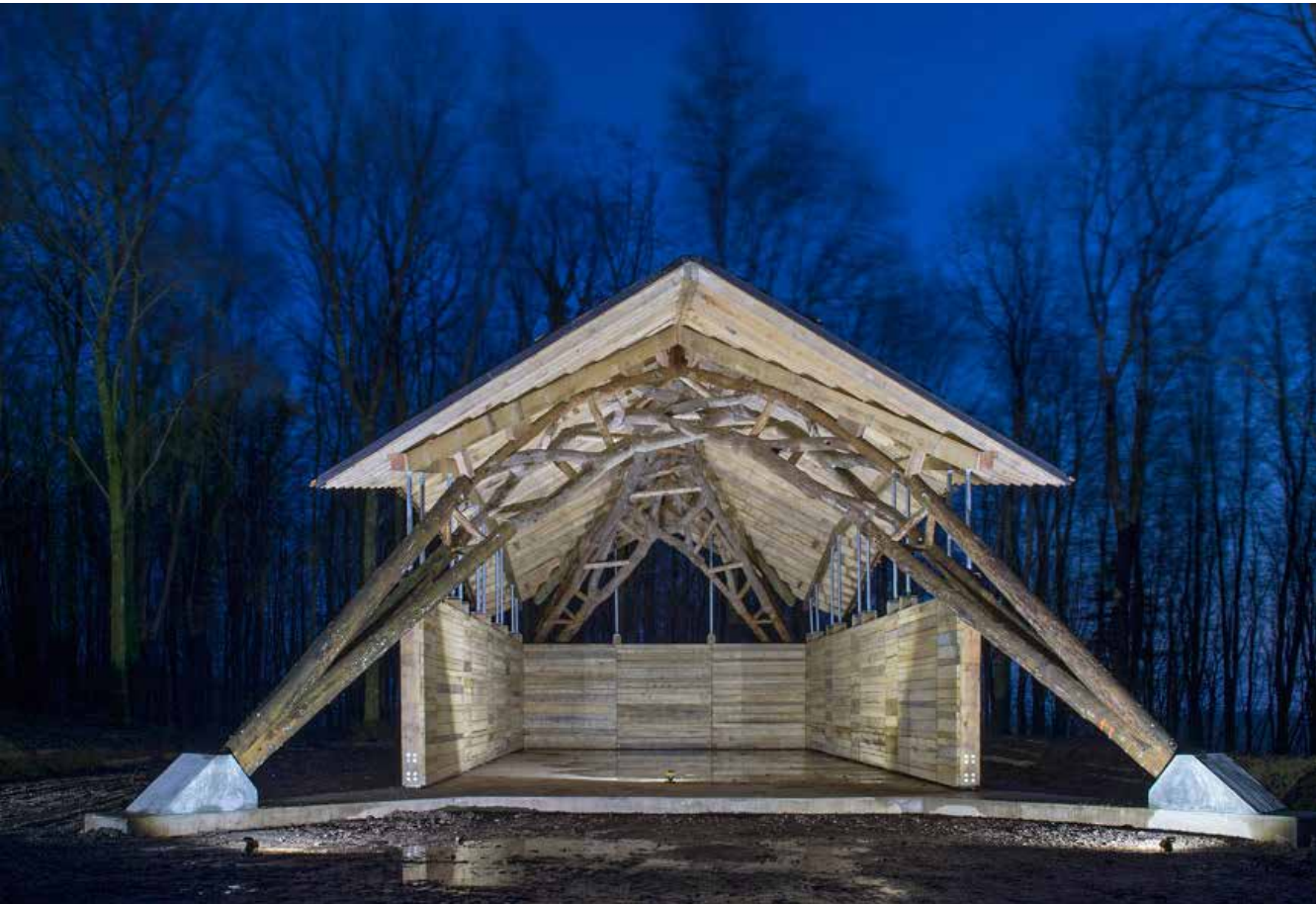
Fig. 5.36 View of the wood-chip barn designed and built at AA Hooke Park using local raw wood. The structural principle is based on the use of tree bifurcations which have been computationally assembled based on their geometric and structural characteristics.
