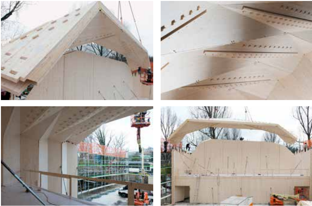
Fig. 5.32 Top: construction process of the theater pavilion on site. Bottom: interior view of the roof after the assembly of the structural elements; the through-tenon connections remain visible in the final construction
