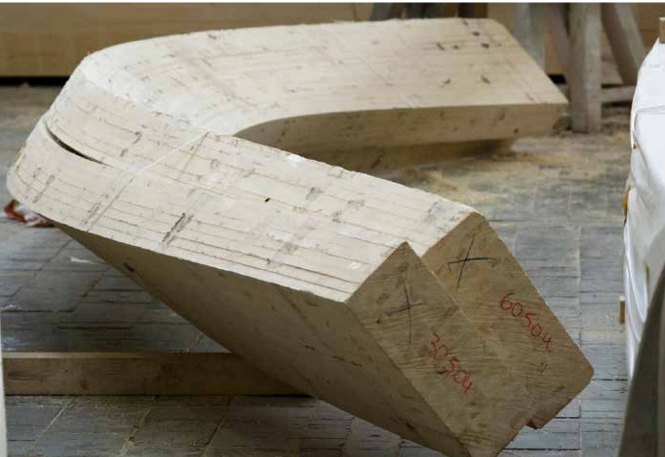
Fig. 5.23 Detail of the double curved timber beams employed in the Centre Pompidou Metz
