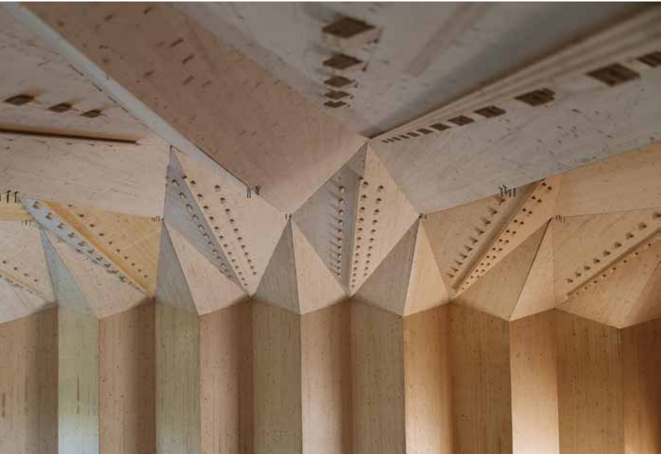
Fig. 5.32 Top: construction process of the theater pavilion on site. Bottom: interior view of the roof after the assembly of the structural elements; the through-tenon connections remain visible in the final construction
