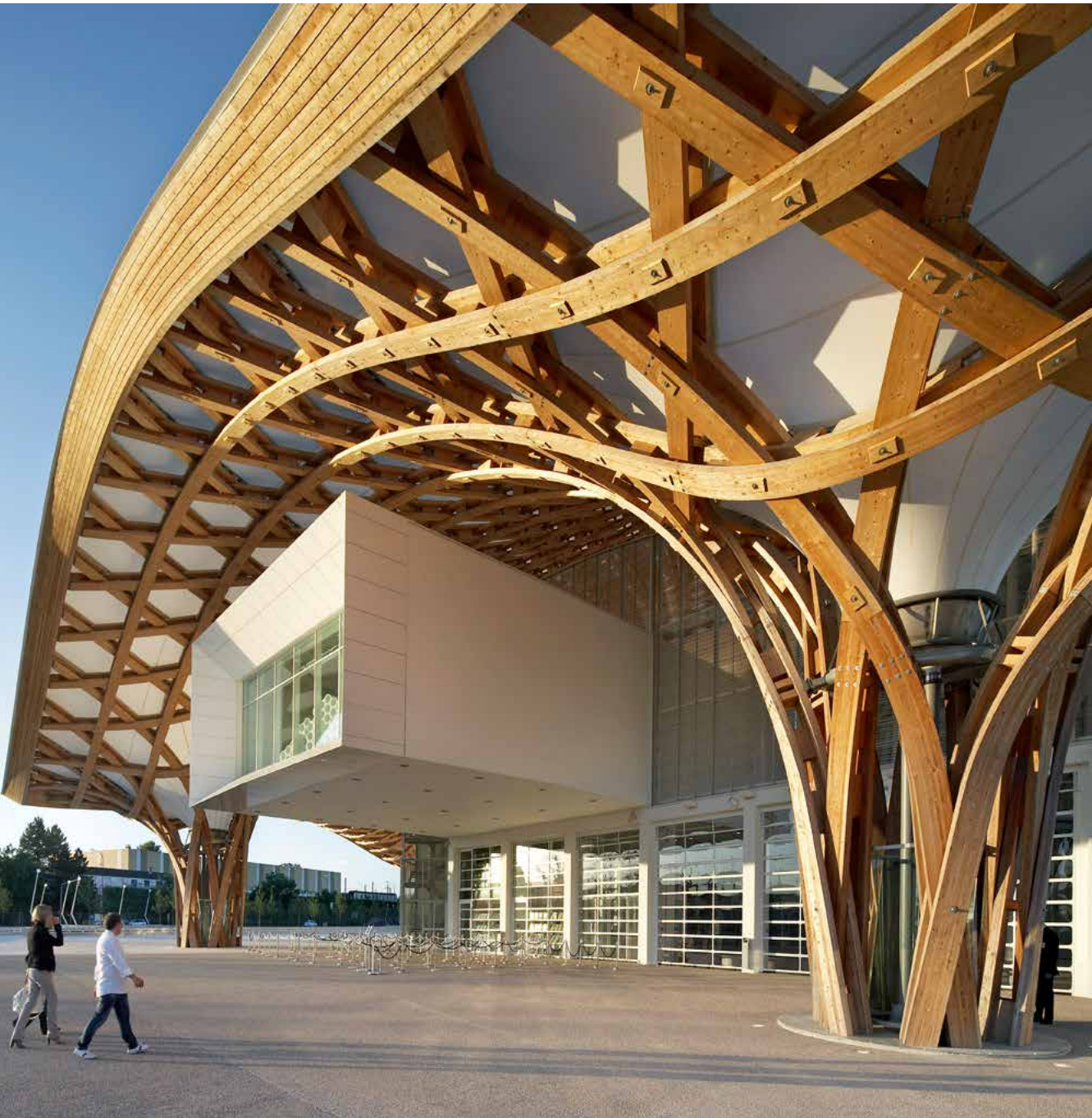
Fig. 3.3 Detail of the timber double-layered structure of the Center Pompidou Metz which has been processed by robots to achieve a curvature of each element in two directions
