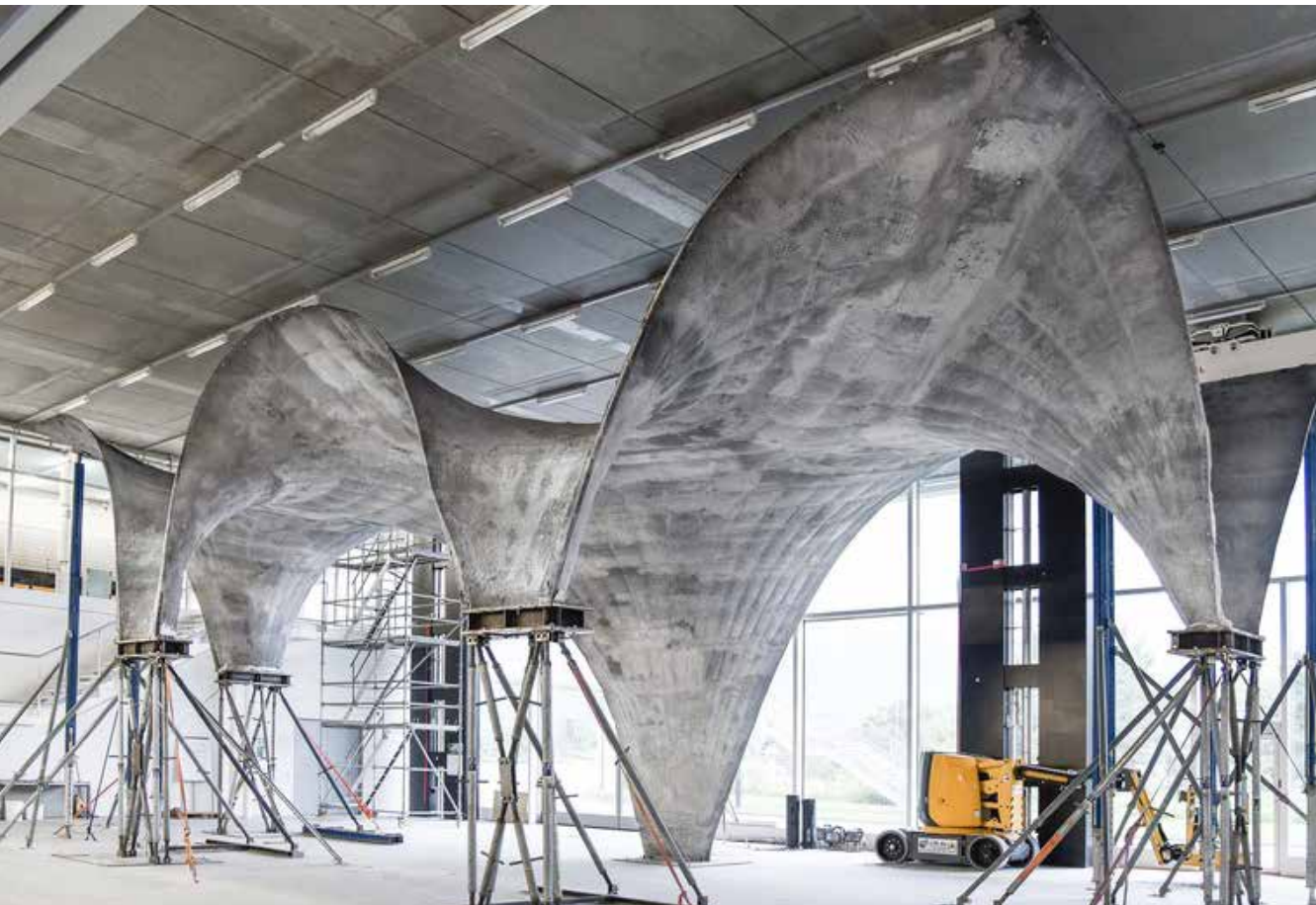
Fig. 2.9 Ultra thin concrete shell for the roof prototype of the NEST-Hilo house, an experimental project by Block Research Group of Zurich ETH
