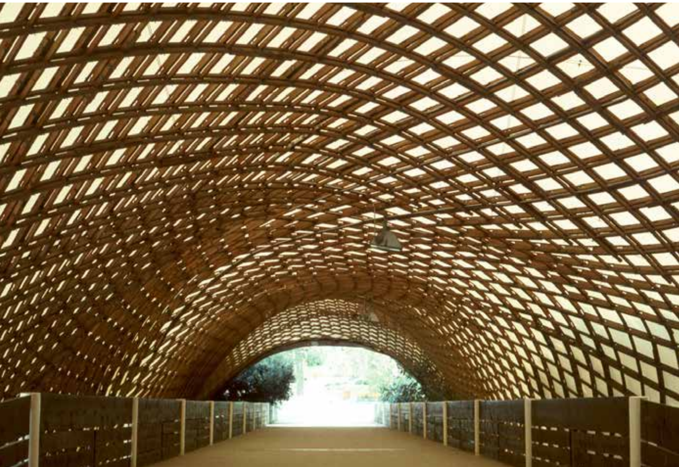
Fig. 4.4 Interior view of the Multihalle that shows the quadrangular grid layout and the double layer.
