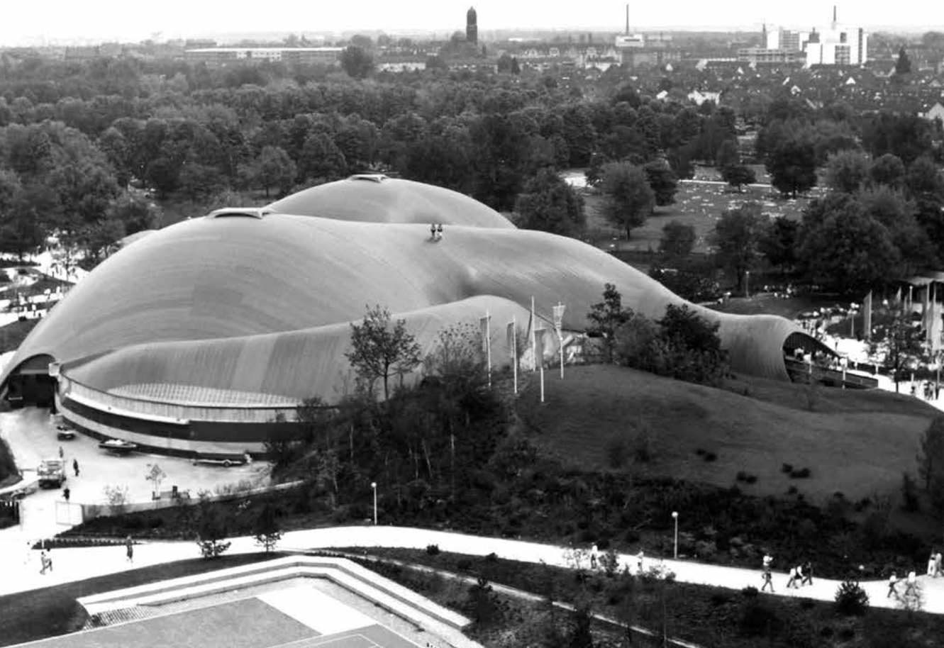
Fig. 4.6 Mannheim Multihalle, roof engineered by Frei Otto in collaboration with Ted Happold and Ian Liddle (Ove Arup).
