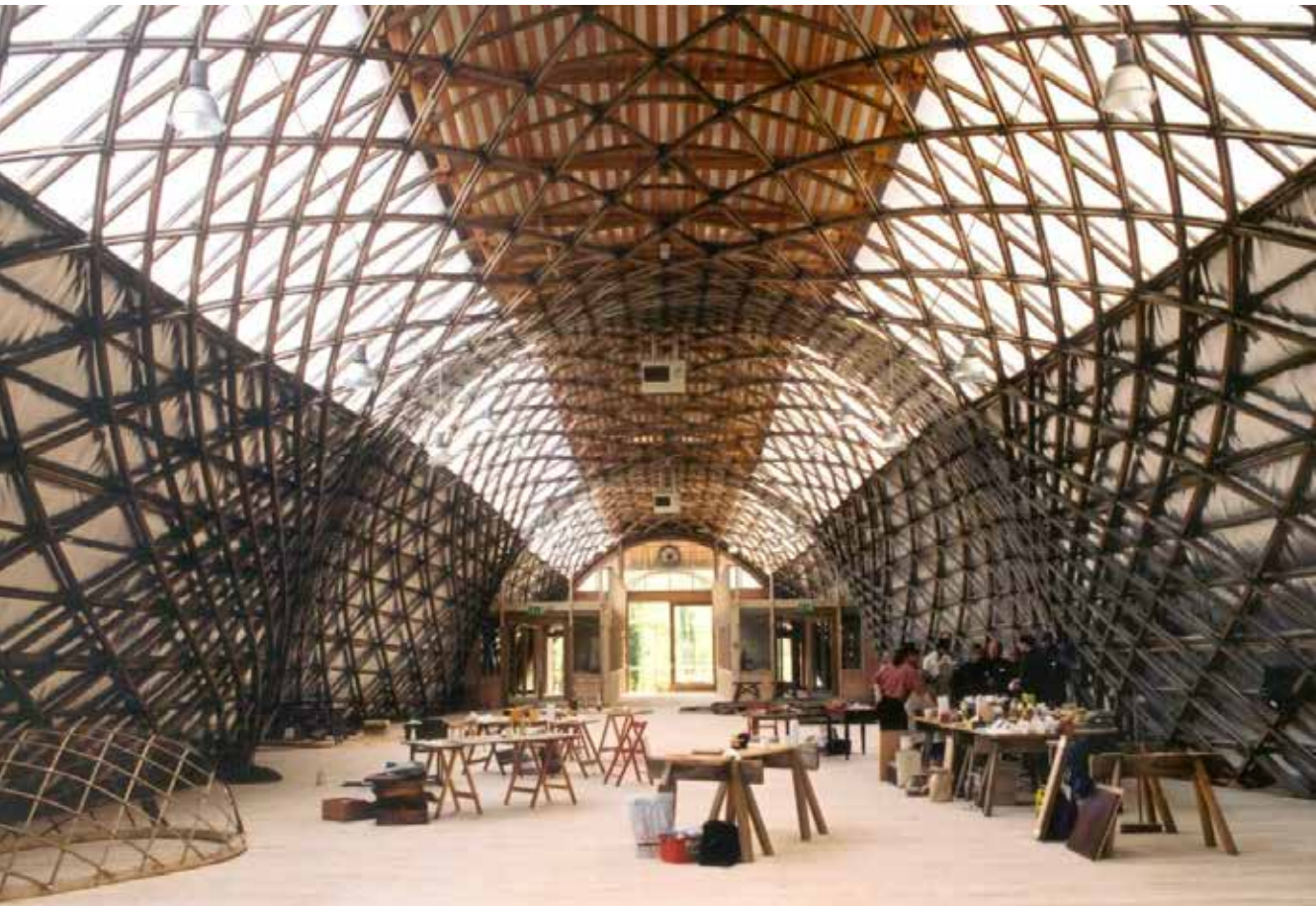
Fig. 4.7 Wealt and Downland wood gridshell by Buro Happold and Edward Cullian Architects. The structural resistance relies on the post-tensioned timber grid, similar to the principles employed in the Multihalle
