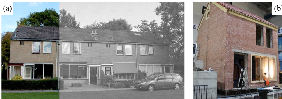
Figure 5.1 a) Front view of a typical Dutch URM terraced house and highlighted end unit and b) overview of the specimen after the construction (adapted from Damiani et al. (2019))
