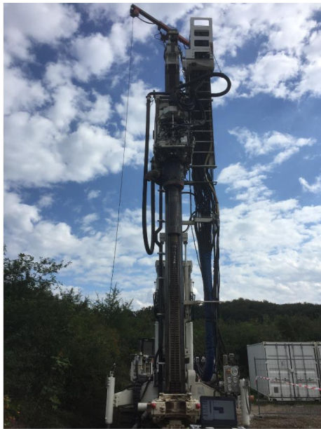
Figure 7: Drilling operations with BO.REX rig.
