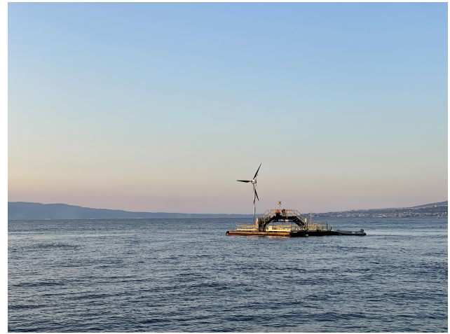
Figure 2. The multipurpose platform.
