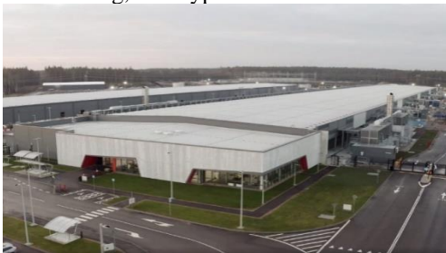
Fig. 1. A typical data centre
