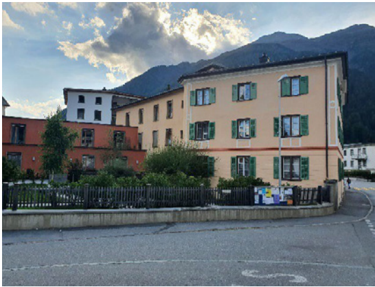
Fig.1: Back-yard of pilot building “Röven 8” F
