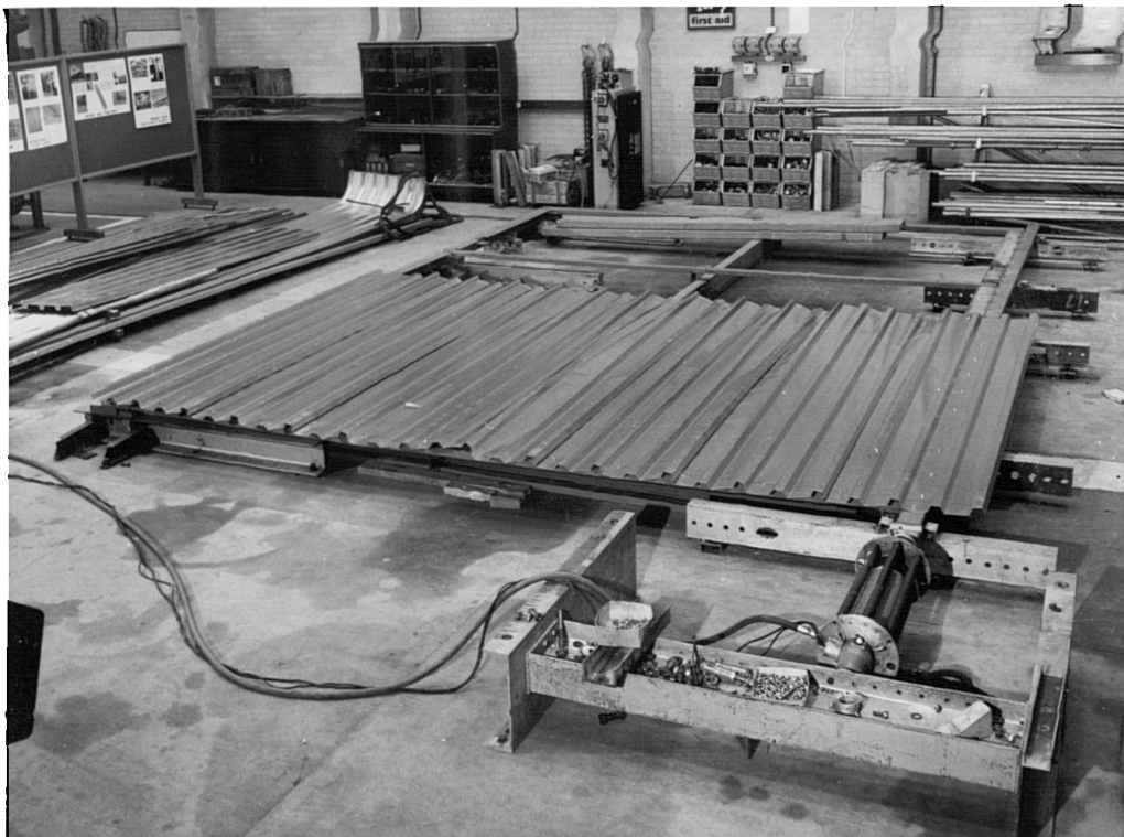
Plate (9.4) Buckling between alternate trough perimeter fasteners
