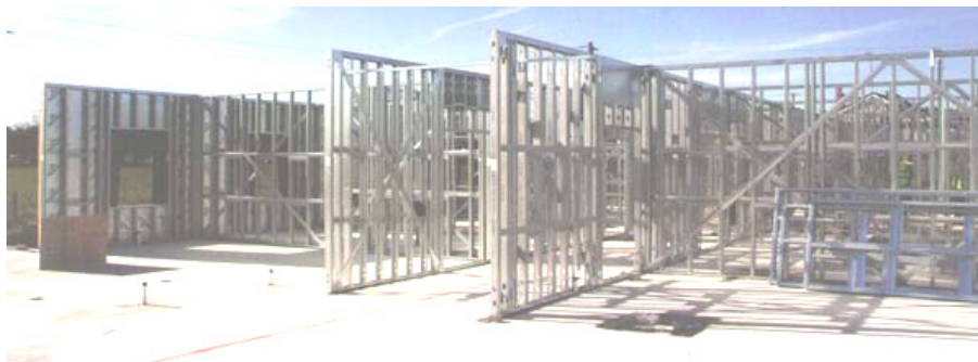
Figure 7: Fixing the steel frames on site (source: Howick, 2010)
