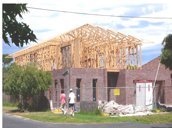
Figure 1: A brick veneer timber framed house under construction
