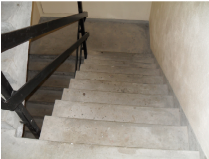
Fig.B3, 4- Typical flight looking down from stair entry point
