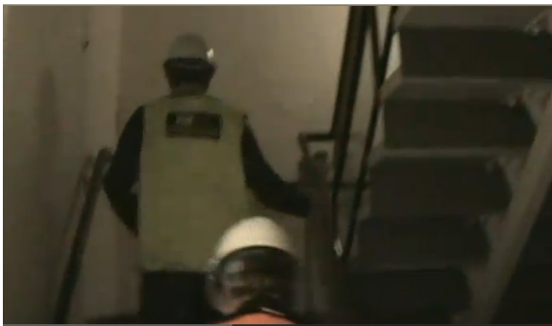
Figure 4-24:- Partial View of Main Fire Stair 123 Victoria Street
