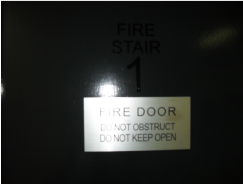
Figure B7.10 - Stair 1 entry door - no contrast for stair number sign above stainless steel warning sign
