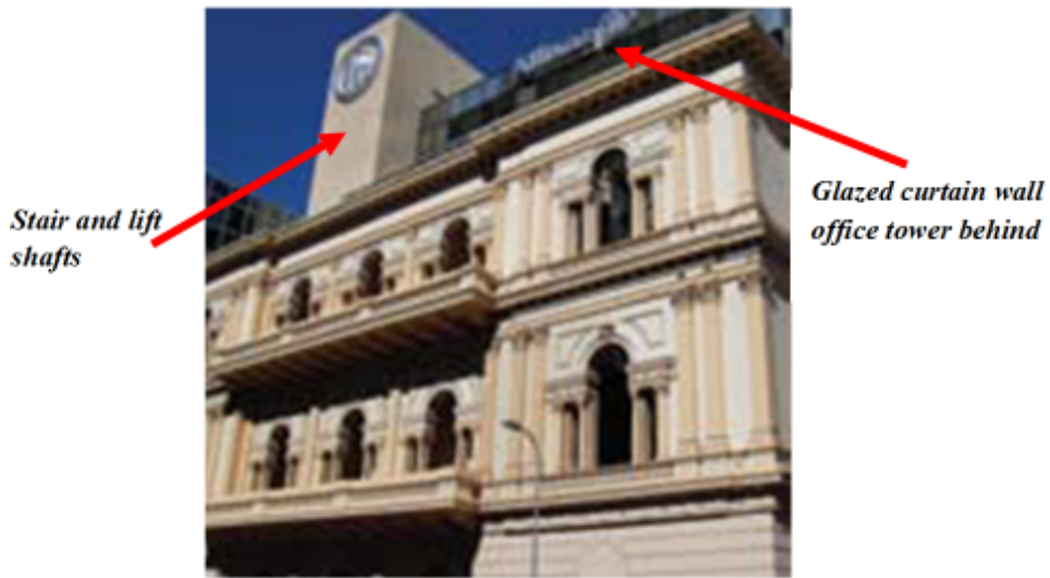
Figure 4-4: Adelaide Building Five – Exploratory Case Study
