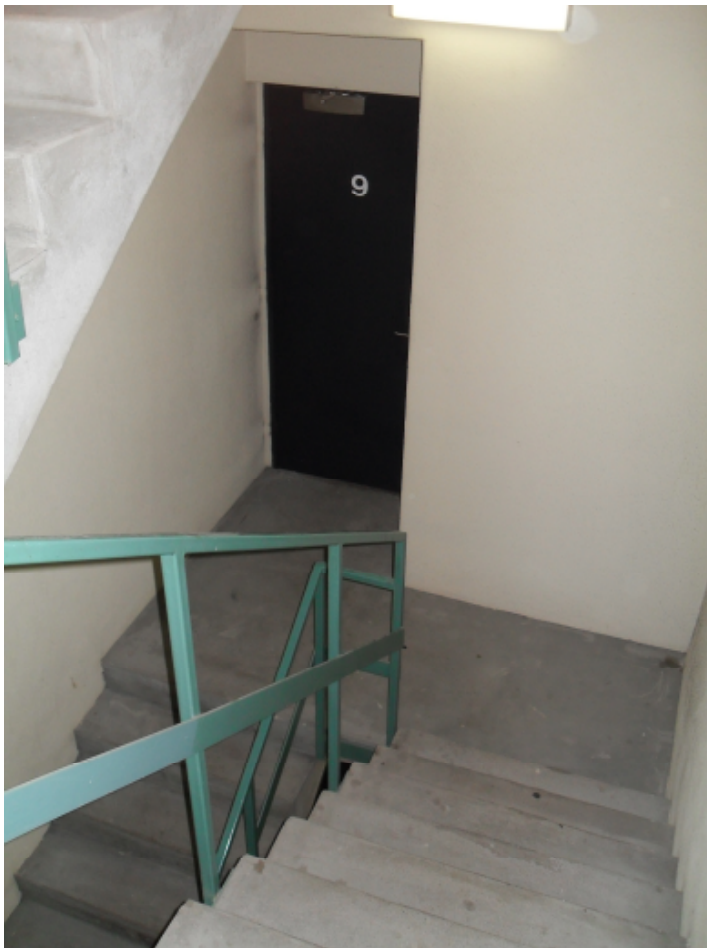
Figure B7.6 - View down typical flight from intermediate landing towards recessed exit access door
