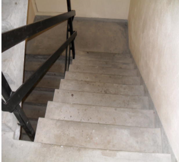
Figure A8: Typical example of handrail rail cross sections - rectangular profile - poor graspability
