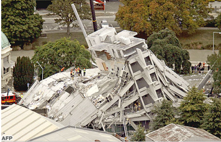
Figure 4-21: Pyne Gould Guinness Office Building
