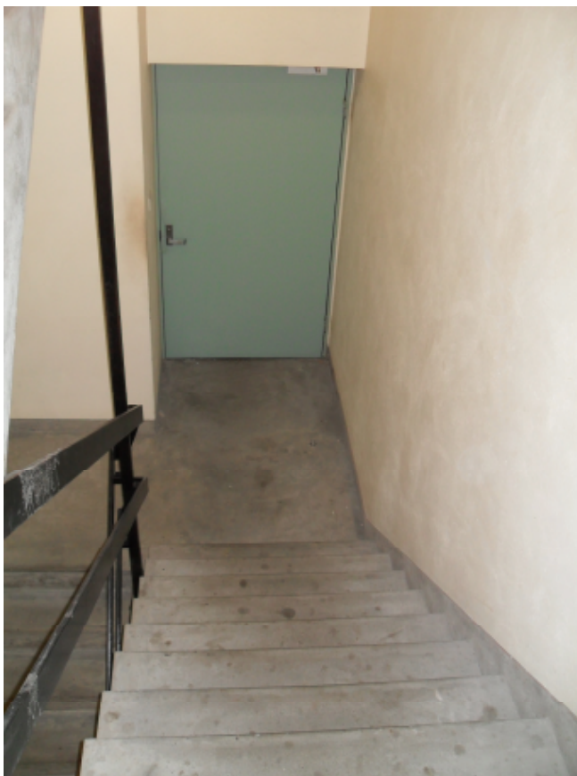
Fig.B3, 6 Looking down flight from intermediate landing to entry door - floor signage not visible
