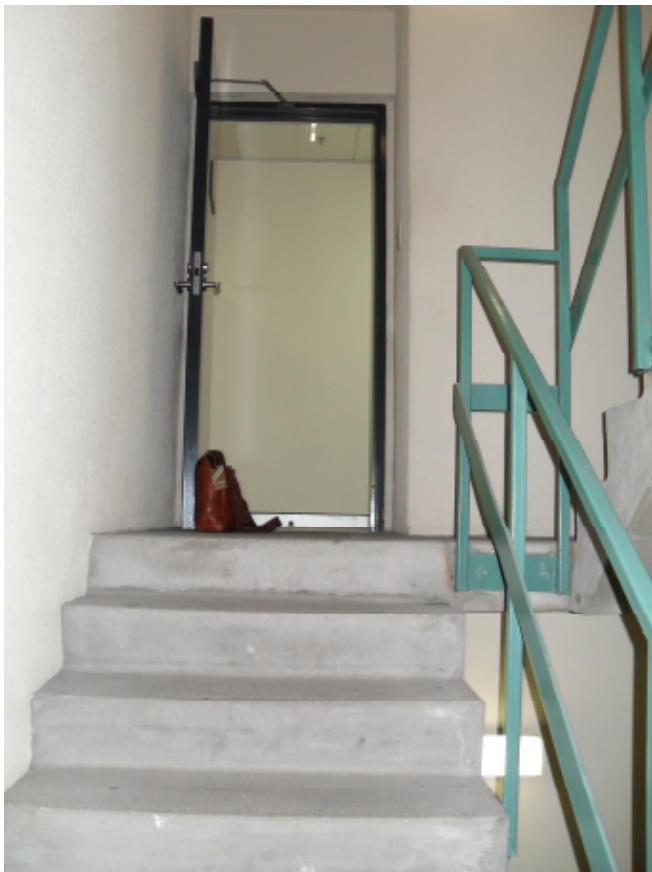
Figure B7.4 - Looking up the down flight towards exit access door
