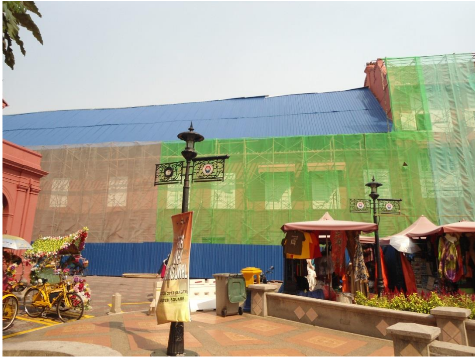
Picture 1: Temporary Roof of the Stadhuys Building.
