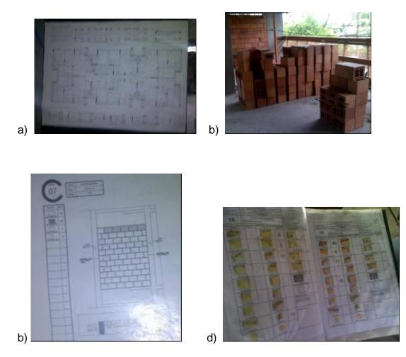
Figure 6.25 (a)-(d): Visualisation of brick laying process and JIT material delivery
