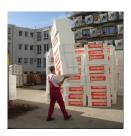
Figure 4.2(d): Storing large amounts of material onsite led to extra work for the construction workers who had to move it about
