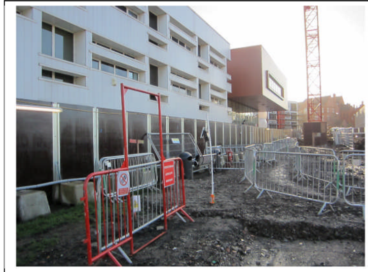
Figure 7-3 Waspmote Installed on Site
