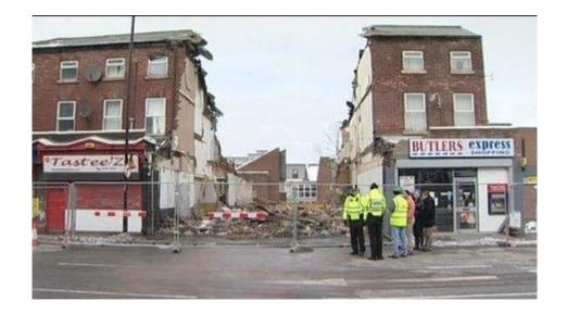
Figure 2-10 Sheffield building collapse blamed on digger (BBC, 2013)
