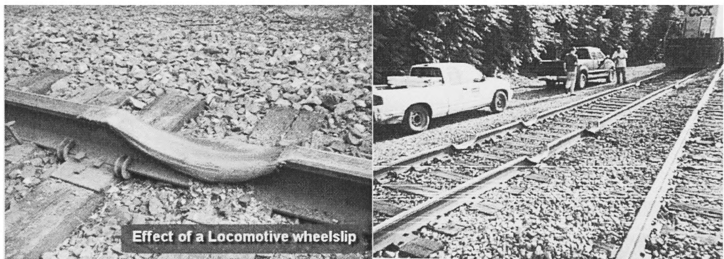
Figure-1.2: Damaged track after severe wheel slip
