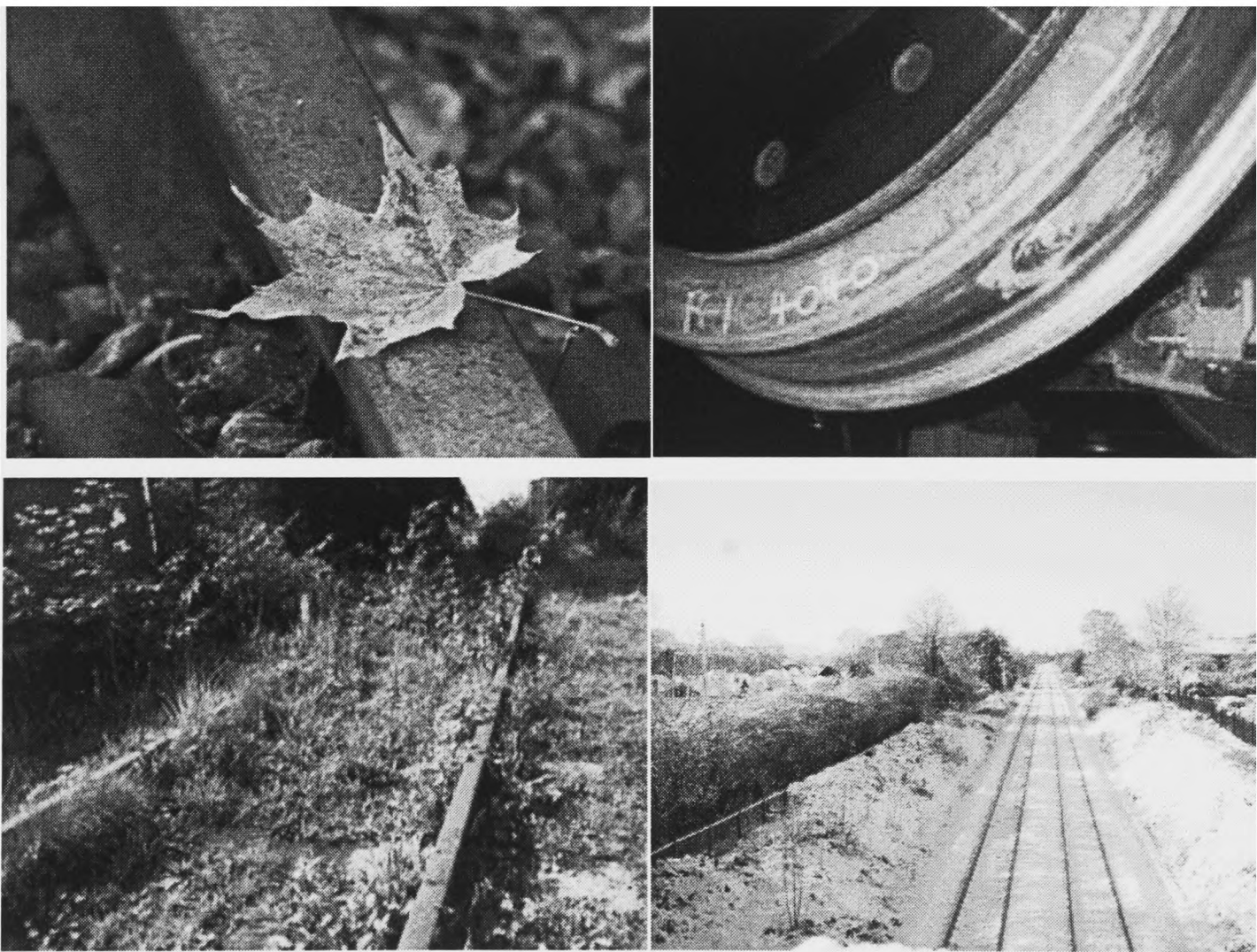
Figure-1.1: Contaminants on railway tracks
