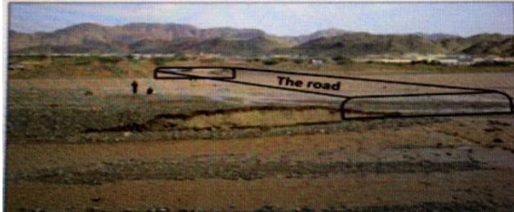
Figure 12.3: Road cut by torrents
