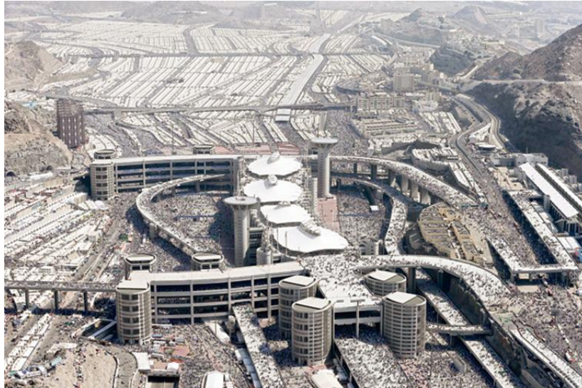
Figure 7.12: The new Al Jamarat Bridge (Source: King Abdul Aziz Public Library, 2012).
