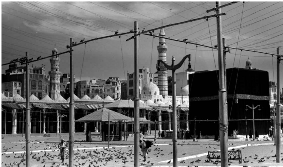
Figure 7.2: The Holy Mosque undergoing repairs under the orders of King Abdul-Aziz in 1947 (photograph by Mohammed Helmi) (Source: Helmi, Mirza, and Bek, 2012,20).
