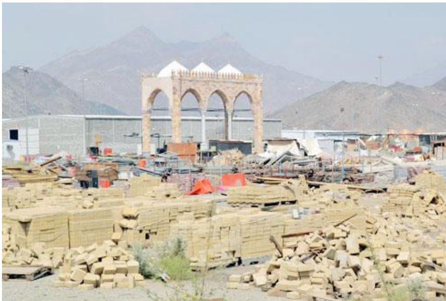
Figure 7.5: A dismantled section of the Ottoman portico awaiting re-installation (Source: Alamadoahi, 2014).
