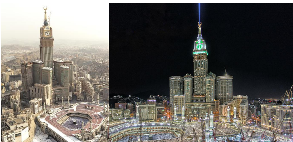
Figure 9.9: Images of Abraj Al Bait Towers after completion (Source: SL Rasch GmbH n.d.)
