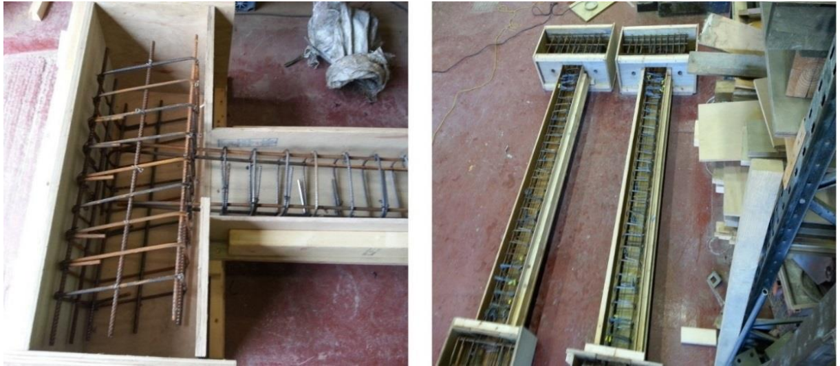
Figure 3-12 Steel Cages with Wooden Moulds
