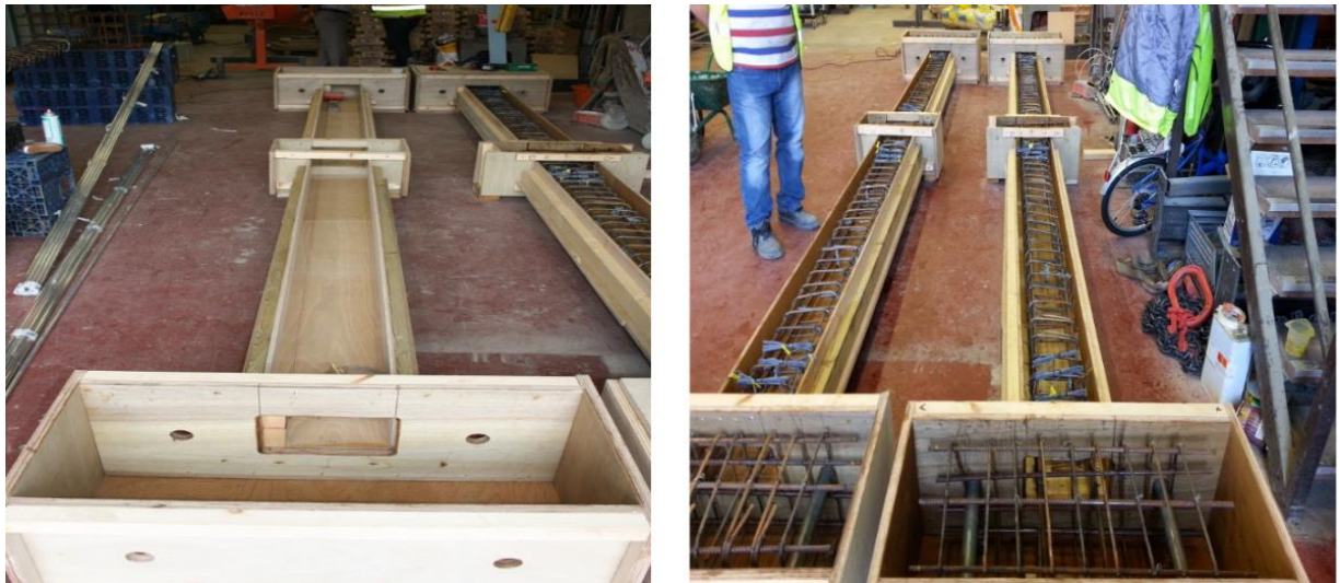
Figure 3-11 Wooden moulds used for concrete casting
