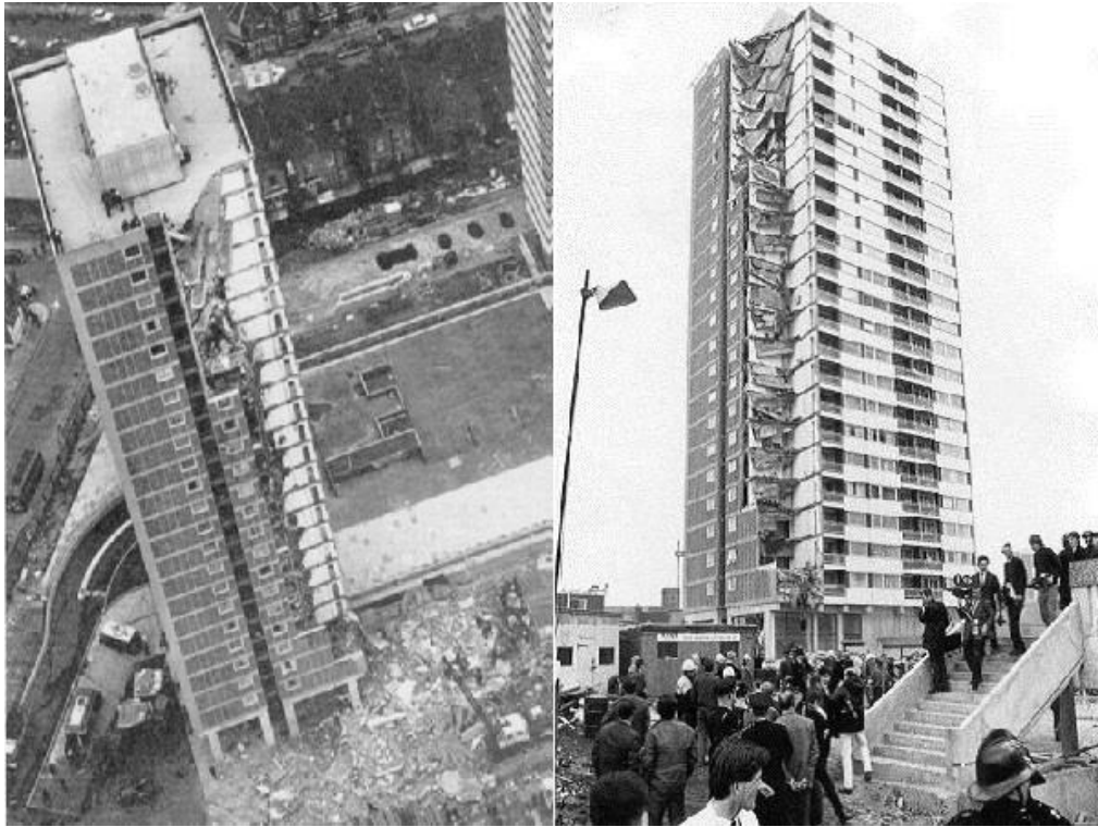
Figure 1-1 Ronan Point collapse (Nair, 2004)
