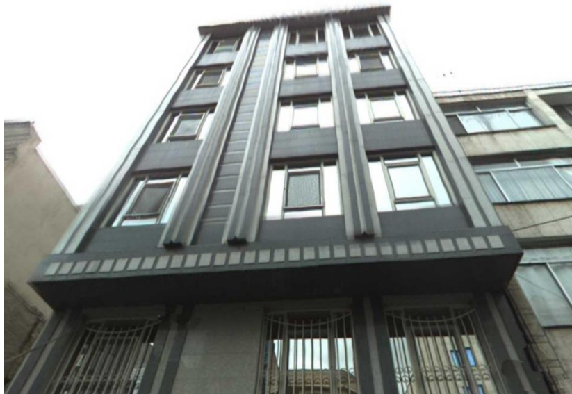
Figure 5.10 – Image of the Actual Building
