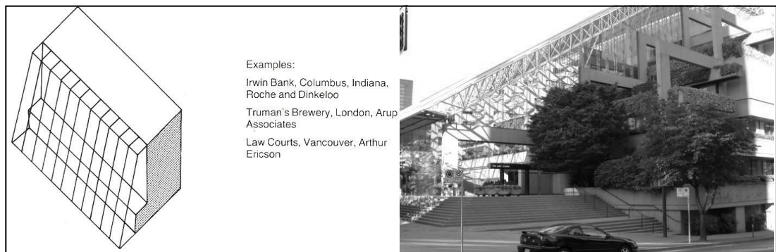
Figure 4. 8: Generic form of a one-sided atrium building on the left (Saxon, 1986) with Law Courts, Vancouver as a one sided example on the right (Halbauer & Company, 2009)
